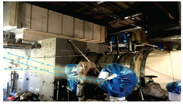
Figure.5: Data transmission between optical wireless field instruments (OWI) and OAP.
