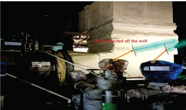
Figure.3: Data transmission between optical wireless field instruments (OWI) and OAP.
