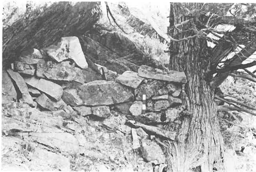
Figure 2: 48TE1076 from south. Note rocks anchored against juniper tree. East wall of structure is directly behind tree. Scale = 25 cm.
