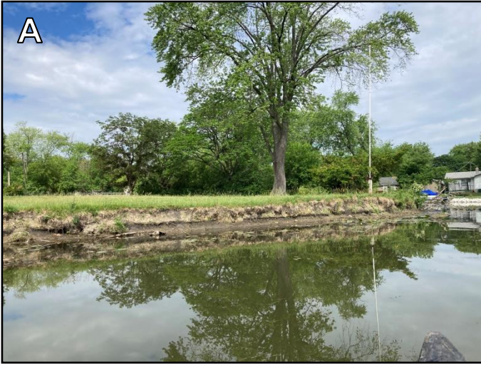
Photo 7. Channel erosion.
