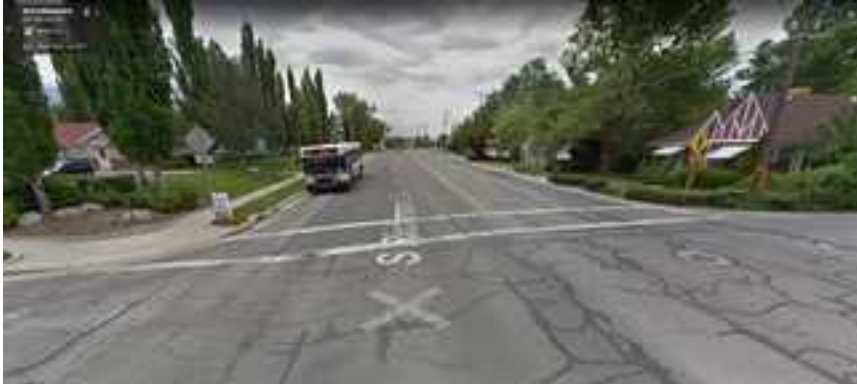
Above: At the intersection of Richmond and Elgin Avenue, there are numerous issues at the crosswalk. For example: the crosswalk has no traffic control device; the street is very wide and speed limits are high; the west side of Richmond has a poor sidewalk with no raised gutter; Elgin west of Richmond has no sidewalk.
