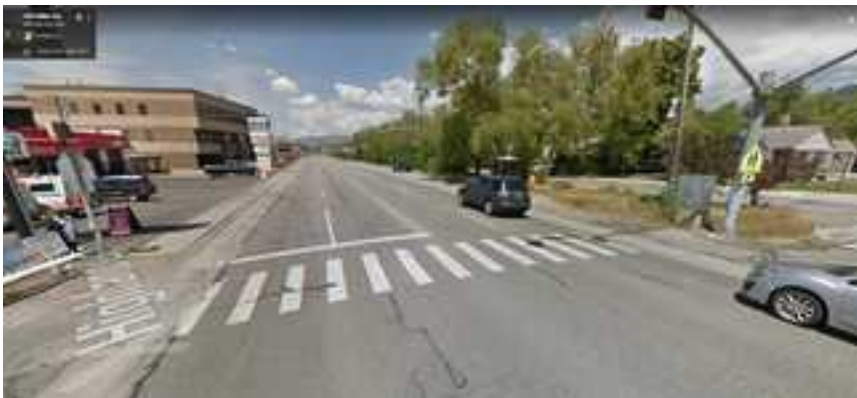
Above: There are several issues at the intersection of Highland Drive and Miller Avenue. These issues include: only two of four sides are crossable for pedestrians; only one of four sides has a traffic signal for pedestrians; and the signalized crossing leads to areas with no sidewalks (the north side of Miller and the east side of Highland lack sidewalks).
