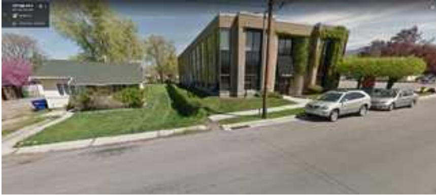
Above: Example of a sidewalk suddenly stopping along Elgin Avenue. The sidewalk, park strip and raised curb/gutter on the right stops at the property line, and an older street design of wide, flat gutter and no sidewalk takes over on the left. The pedestrian is forced to cross over the park strip and then walk in the gutter or the street.
