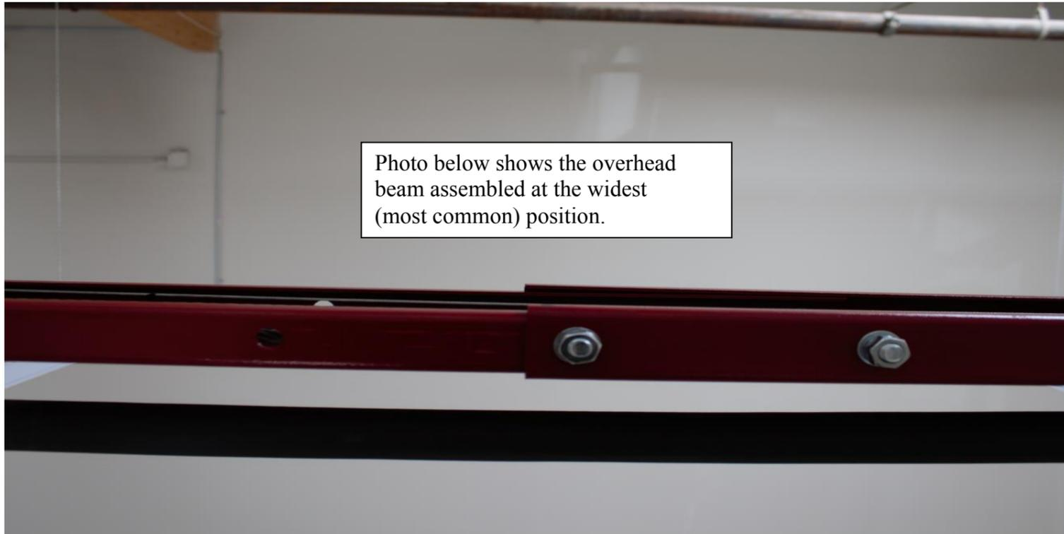
While the overhead beam is still on the shop floor install the provided 4 pulleys (sheaves). Two (2) pulleys on each side of the overhead beam using the parts shown below. Note: Asymmetric installation (rotated column position as shown in figure 5) requires the pulleys to be installed offset to each other using two (2) axles and related parts. Symmetric installation (as shown in figure 4) requires the pulleys to be installed on a common axle using the related parts. *See related photos below.*
