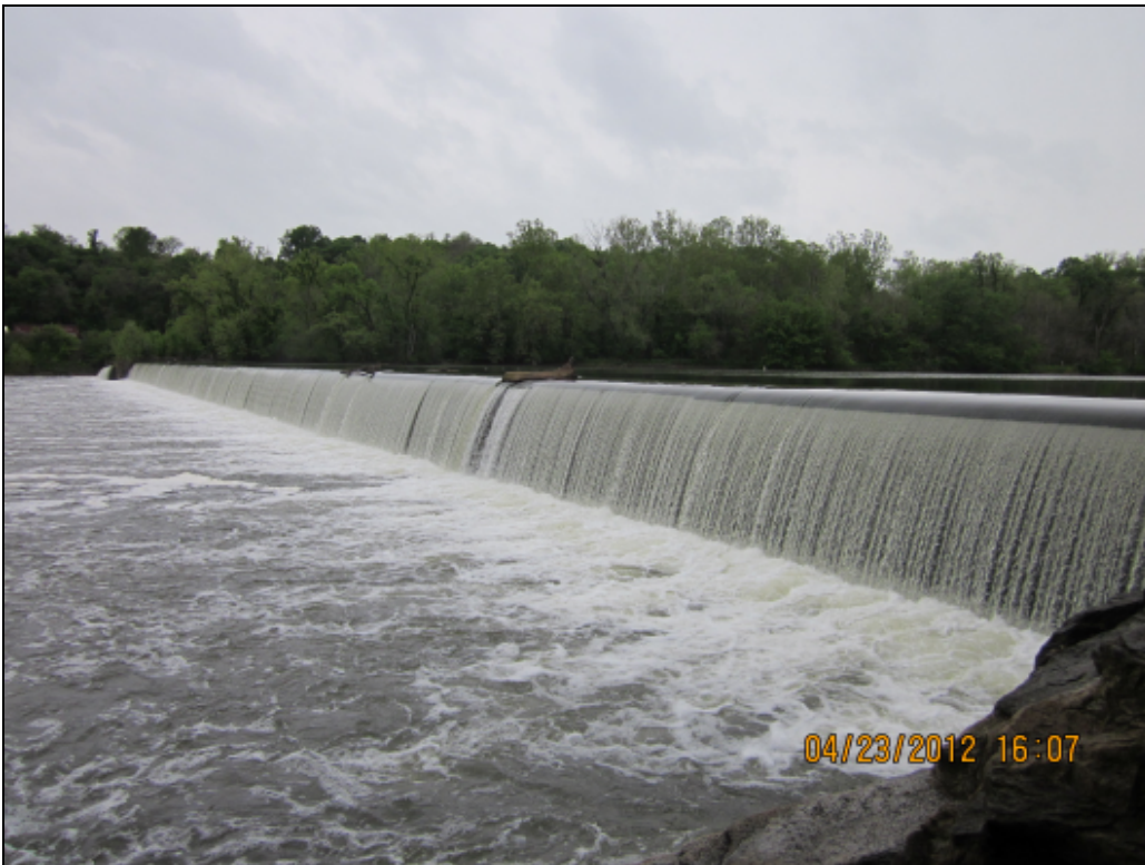
Photograph 2: Straight eastern portion of dam (view west-southwest)
