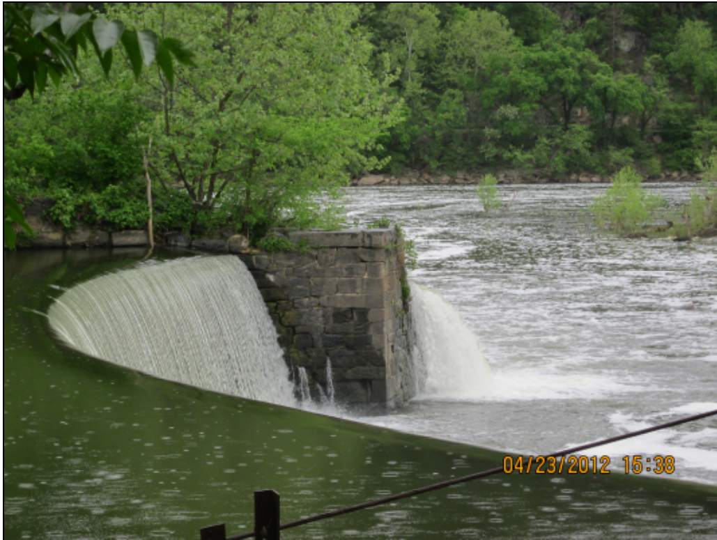
Photograph 1: Arched western portion of dam (view east-northeast)
