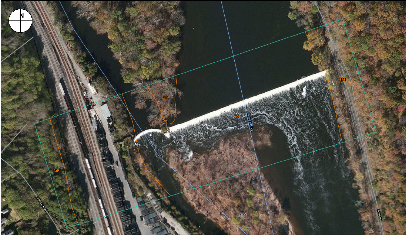
37E – Stott Knob-Rhodhiss complex, 20-50% slopes, very stony Tf – Tallapoosaloam, 25-60% slopes W - Water CT – Chewacla-Toccoa complex UL – Urban Land
