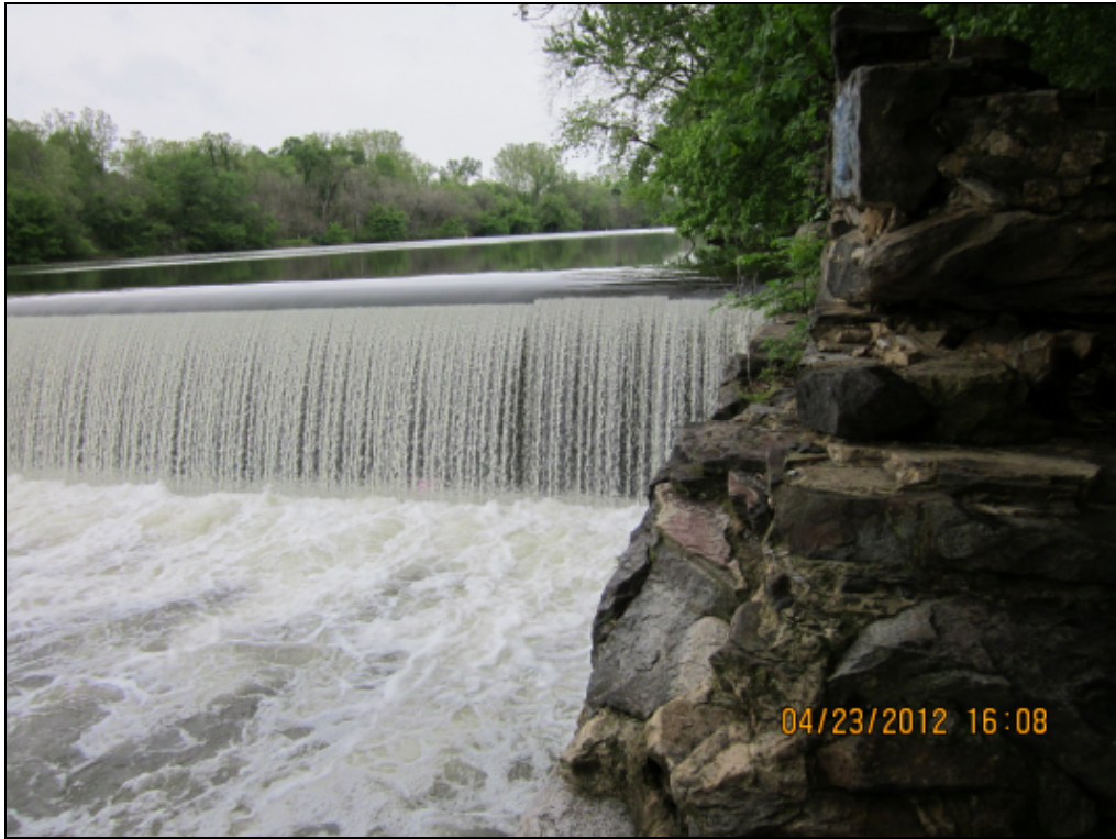
Photograph 5: Relic stonework, eastern terminus of dam, and view upstream (view north)
