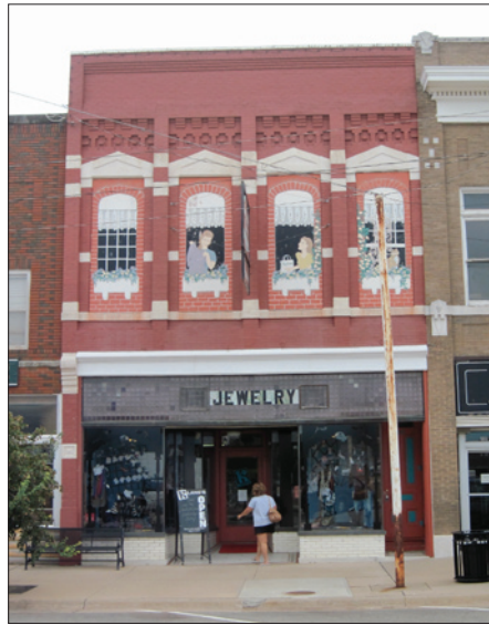
A downtown Anthony building with murals in the areas where there were windows.
