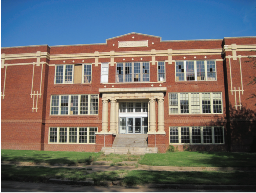
The historic high school sits vacant with broken windows.
