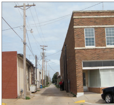
View of alley behind Main Street that carries utilities.
