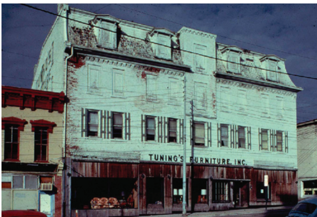
Many communities have large “white elephant” buildings (above) that remain vacant due to obsolete uses. However, many are converted (right) to new uses like this old hotel that is now a community center for history and art.
