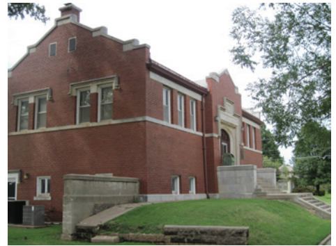
The Jacobethan-style Carnegie Library, listed on the National Register of Historic Places, was built in 1911. It is currently vacant.
