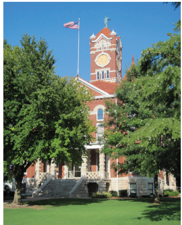
The Harper County Courthouse clocks were undergoing restoration during the site visit thus this image shows plywood in the cupola where the clocks are housed.
