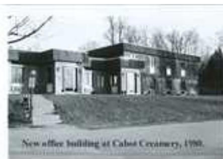
1980's New Office Building: - from the Cabot Historical Society collection.
