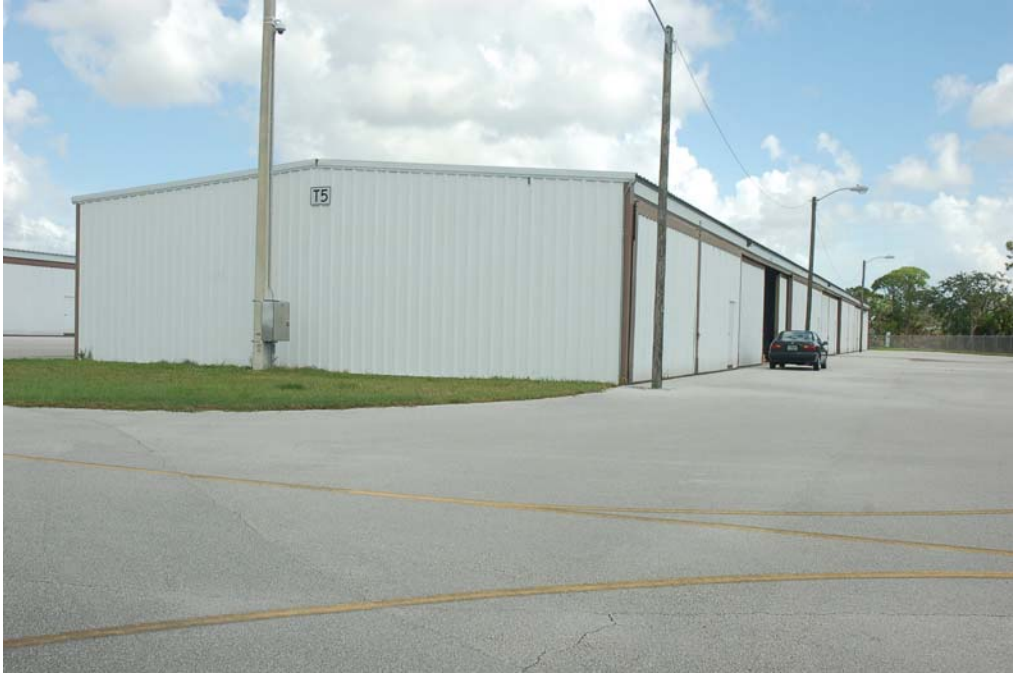
View of the south and east elevations.
