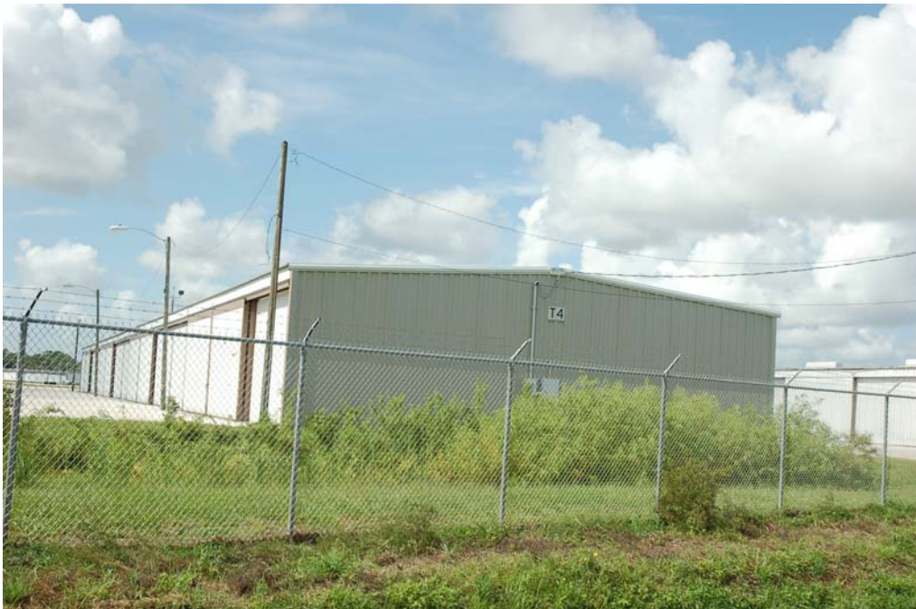
View of the north and east elevations.
