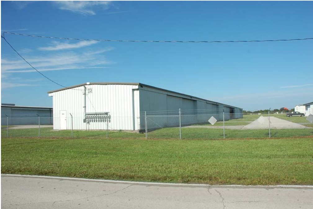
View of the north and east elevations.
