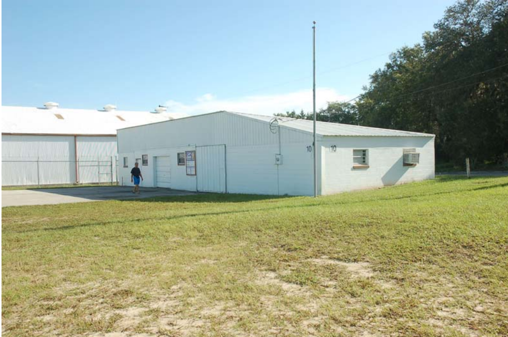
View of the south and west elevations.
