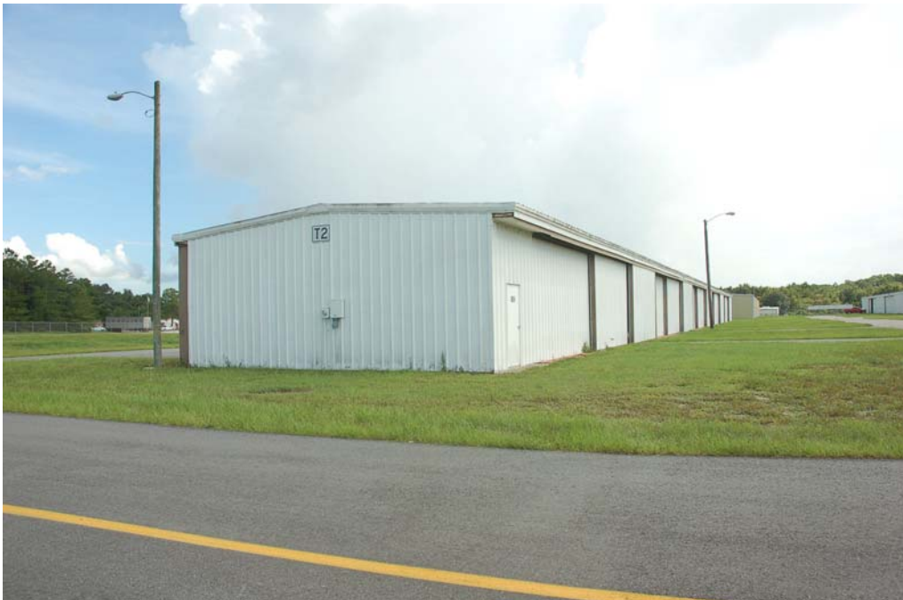
View of the north and west elevations.
