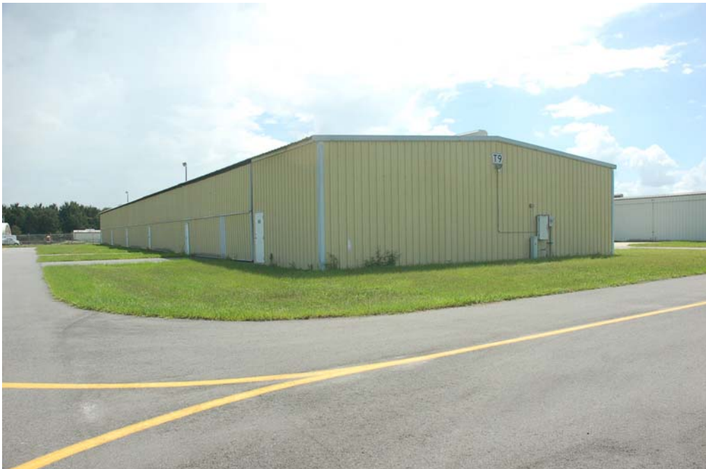
View of the north and east elevations.
