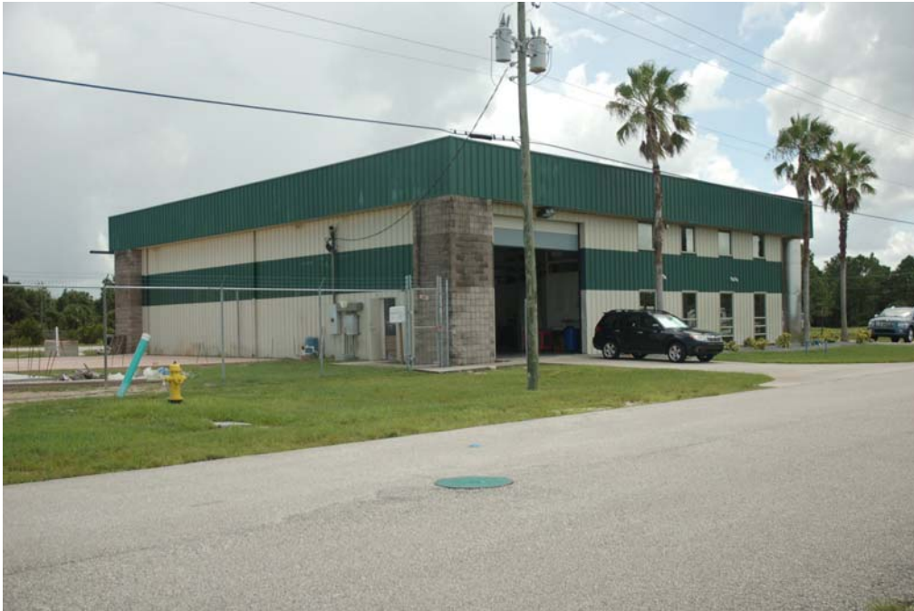
View of the north and west elevations.
