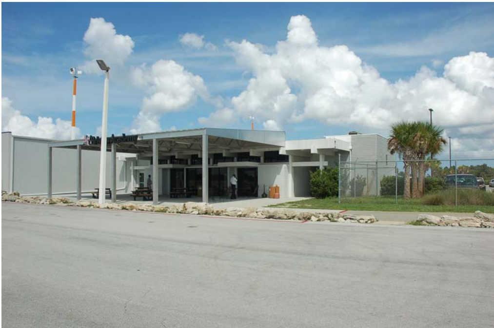
View of the south and west elevations of the original building.
