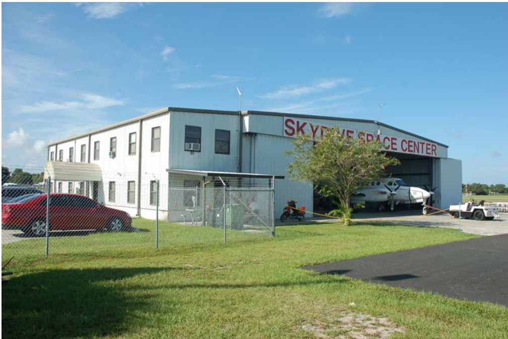
View of north and east elevations.
