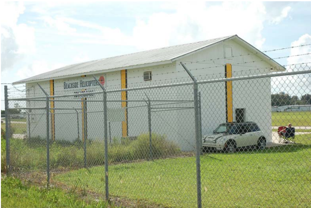
View of the north and west elevations.
