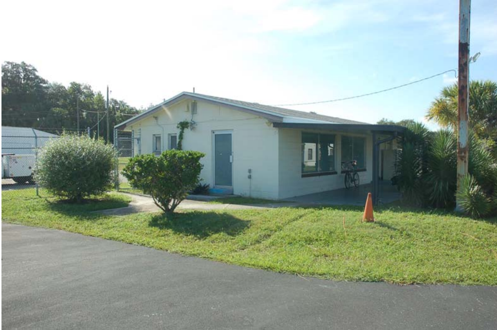
View of the north and west elevations.
