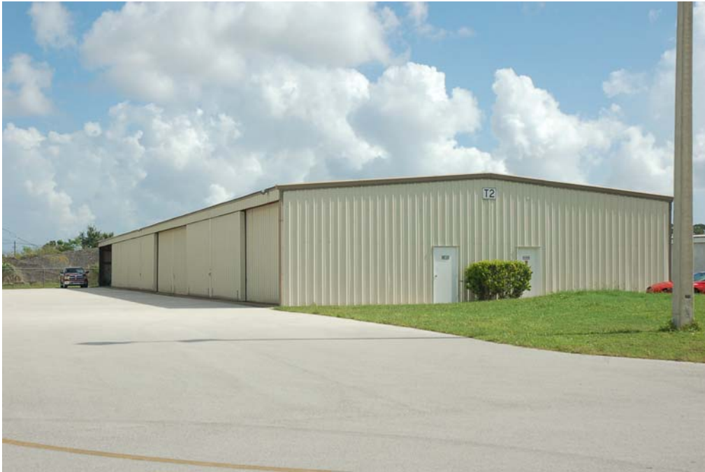
View of the south and west elevations.
