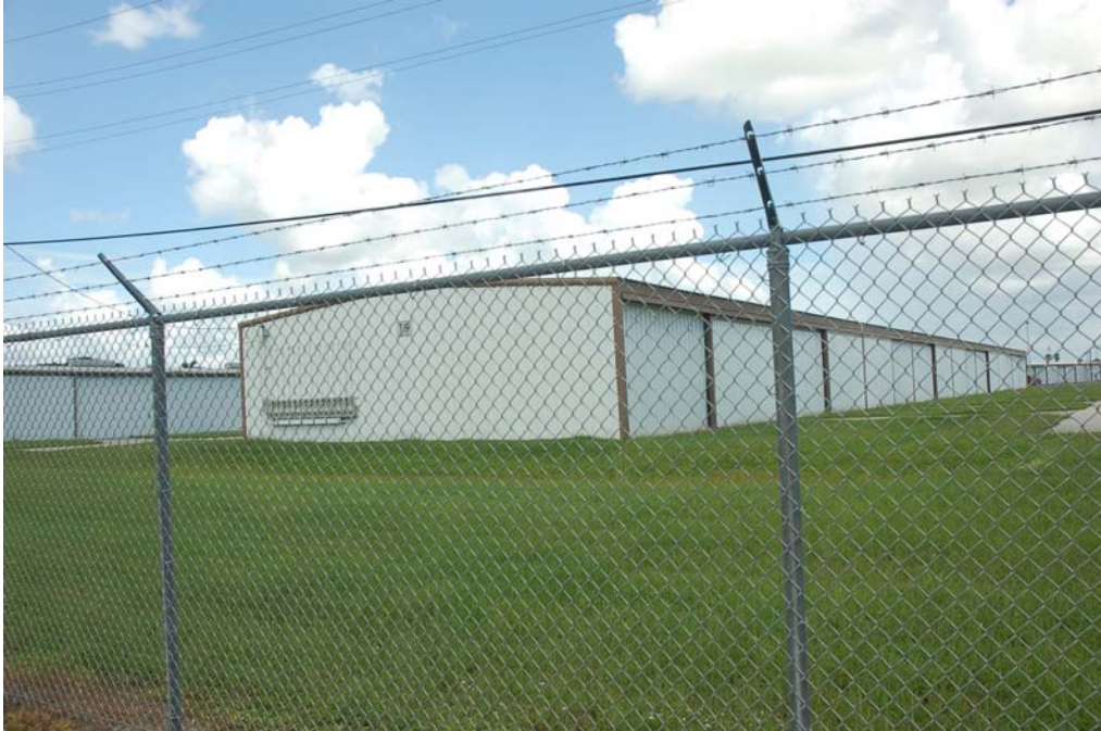
View of the south and east elevations.
