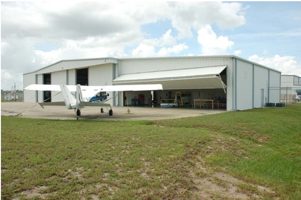
View of the north and east elevations.
