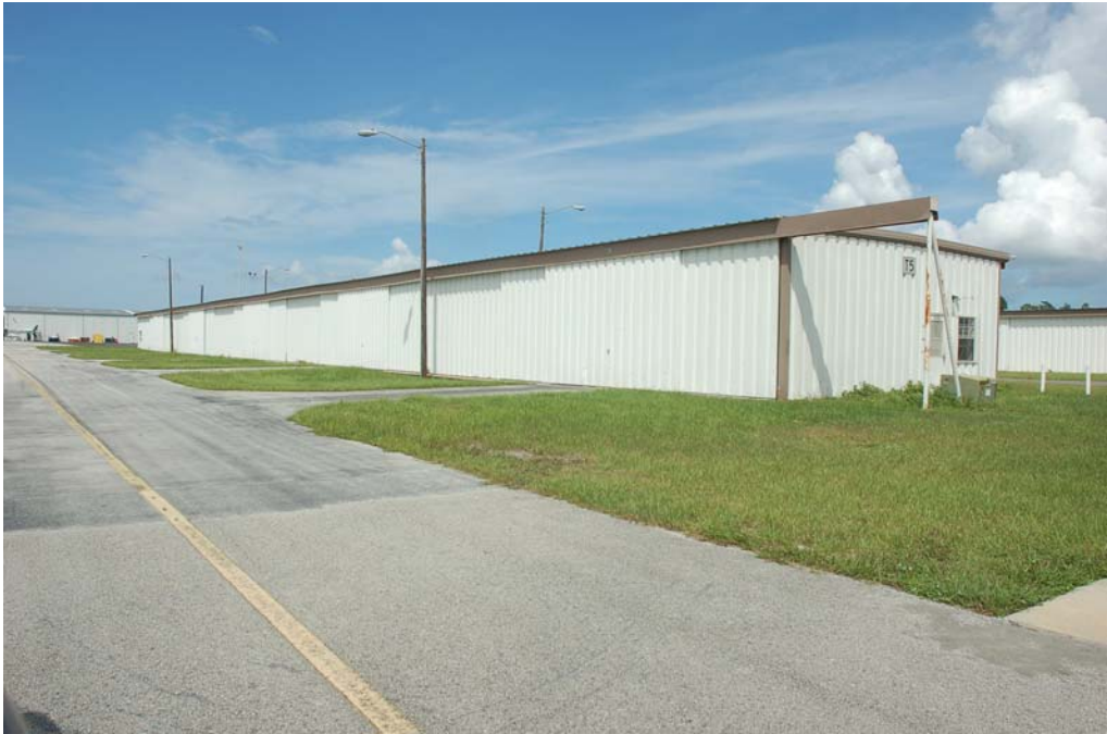
View of the south and west elevations.
