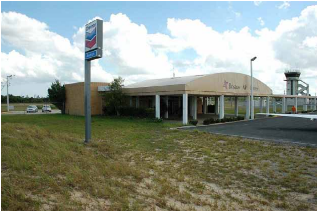
View of the north and west elevations.
