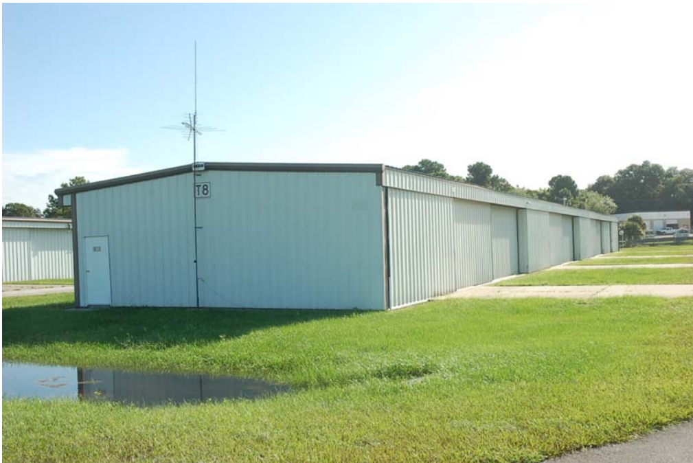
View of the south and west elevations.
