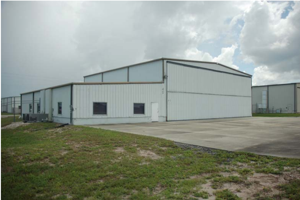
View of the north and west elevations.
