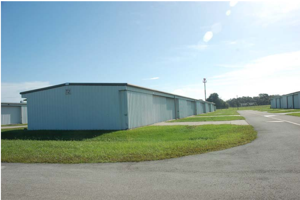
View of the north and east elevations.
