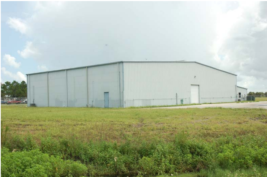
View of the north and west elevations.
