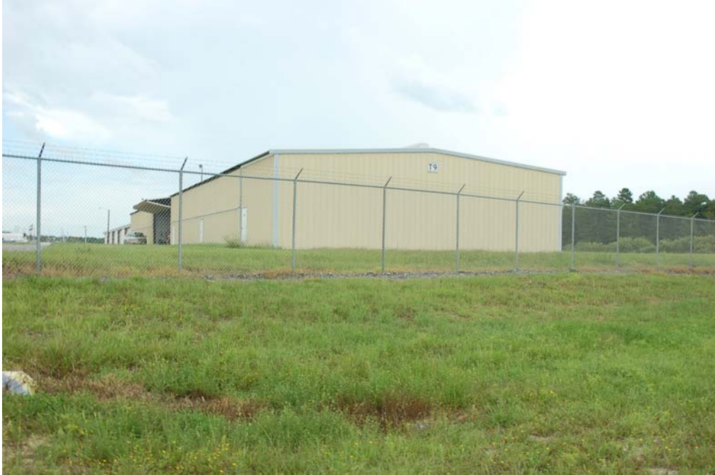
View of the south and west elevations.
