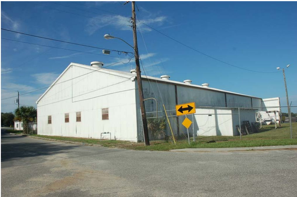
View of the north and east elevations.
