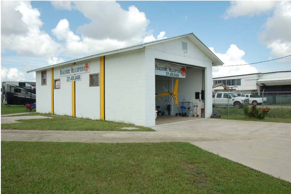
View of the south and east elevations.
