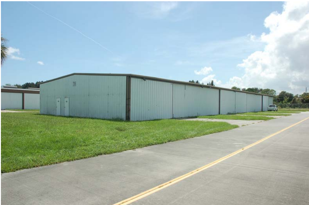
View of the north and west elevations.
