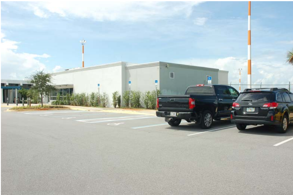
View of the south and east elevations of the new addition.
