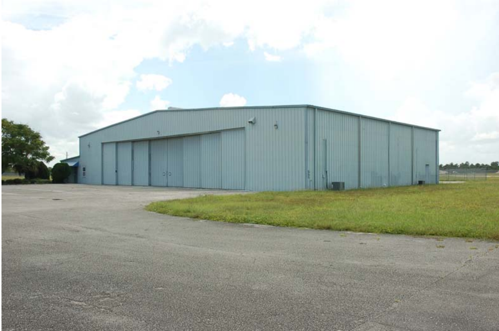
View of the north and east elevations.
