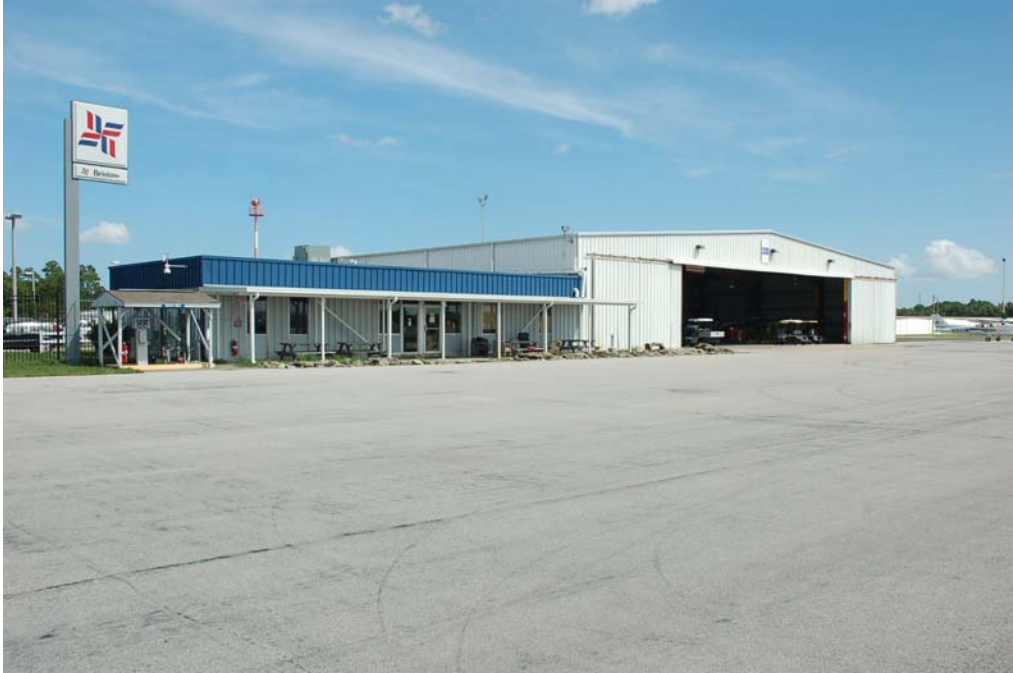
View of the north and west elevations.
