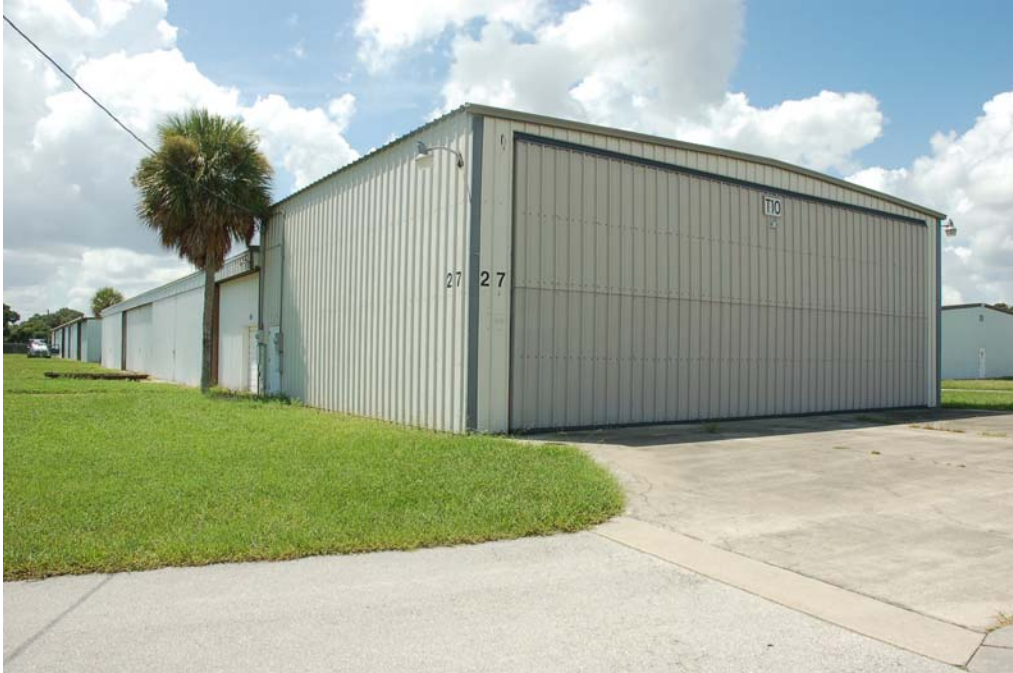
View of north and east elevations.
