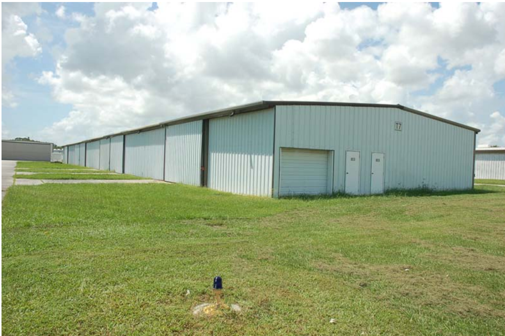
View of the north and east elevations.
