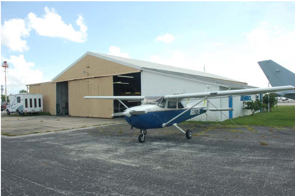
View of the south and west elevations.
