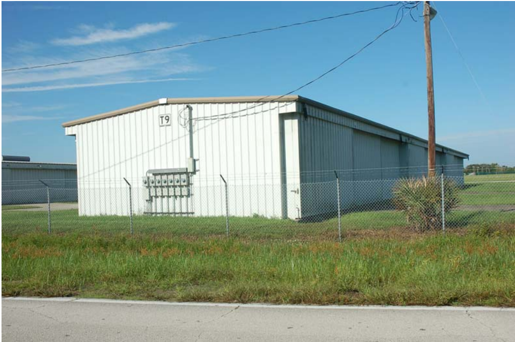
View of the north and east elevations.
