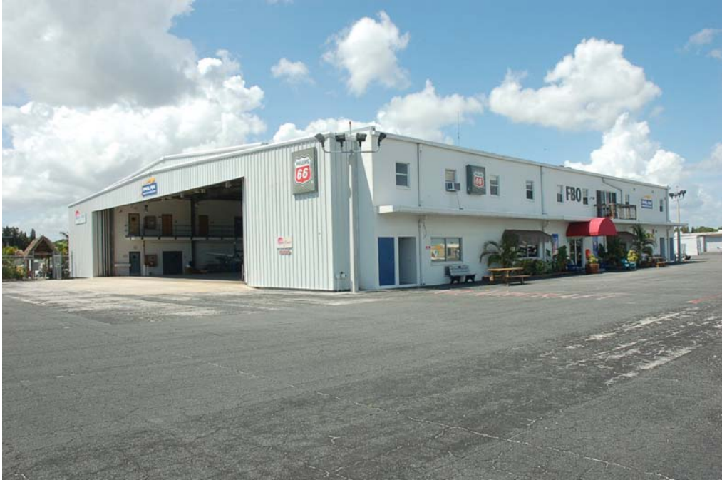
View of the north and east elevations.
