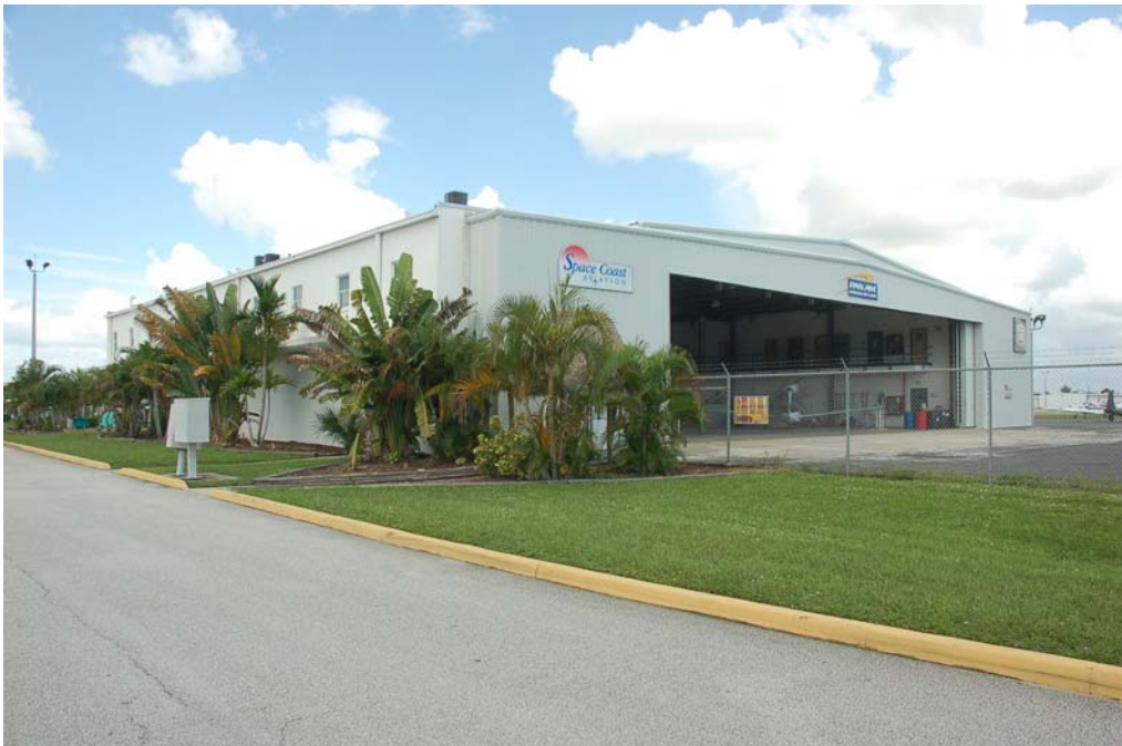
View of the south and east elevations.
