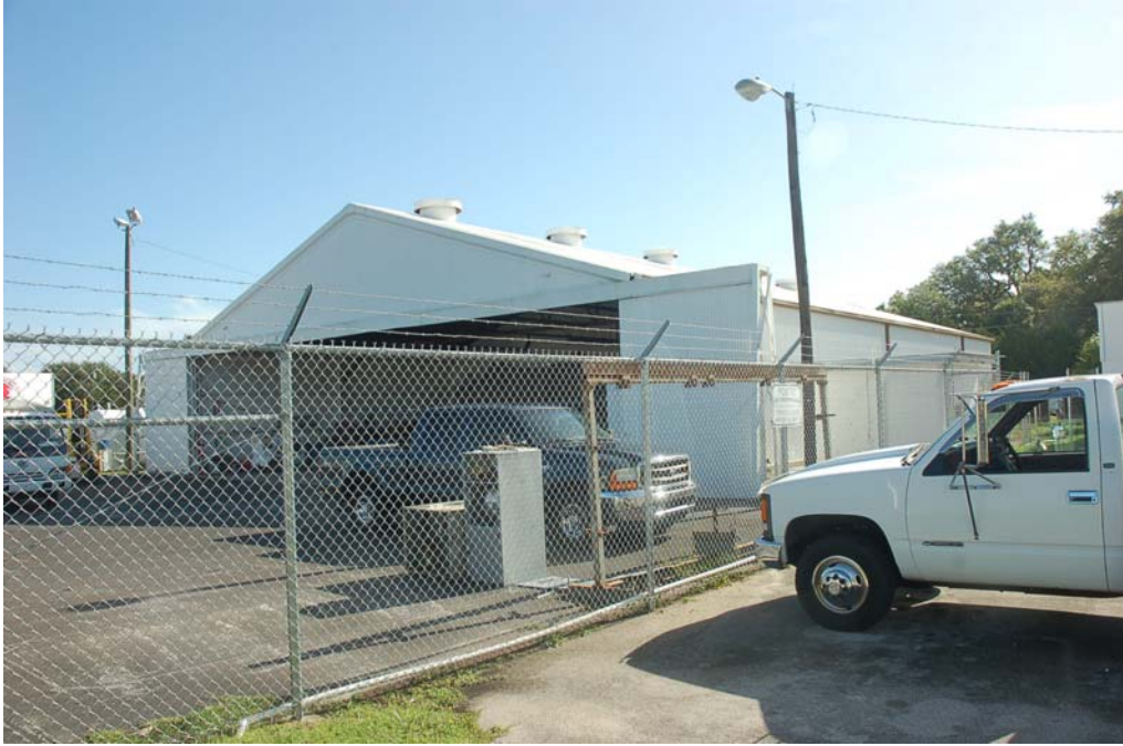
View of the south and west elevations.
