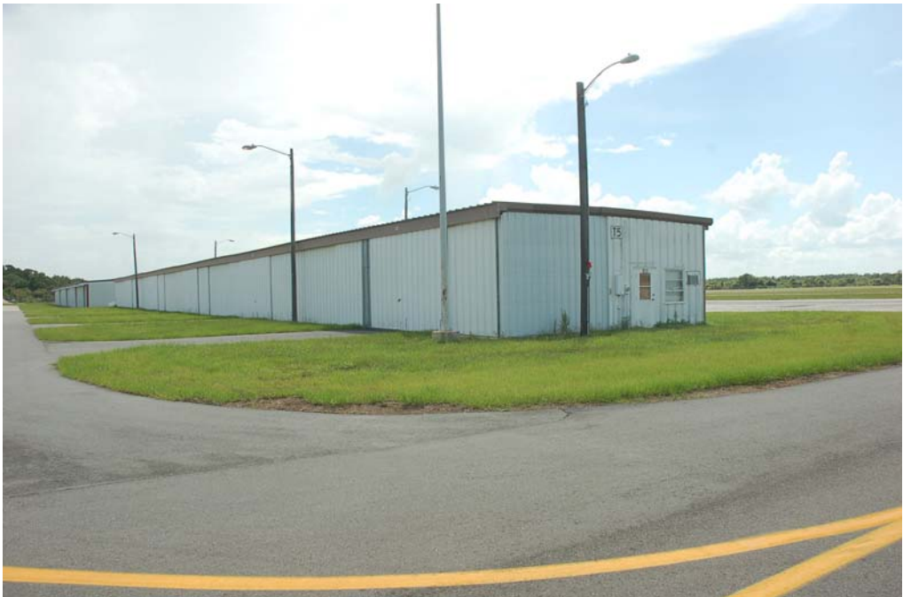
View of the north and east elevations.
