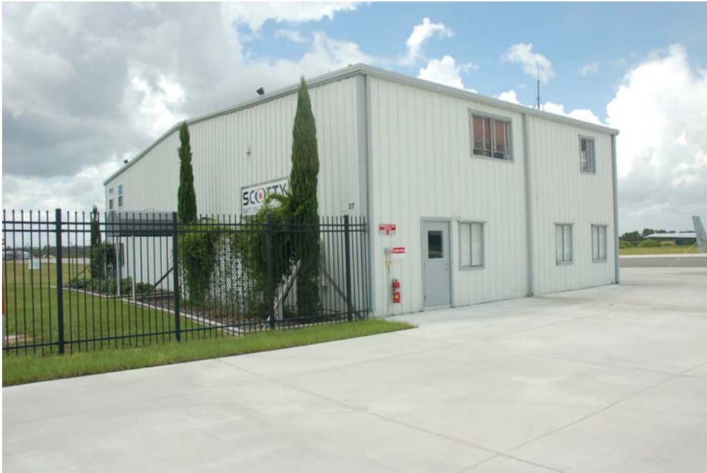
View of the north and east elevations.
