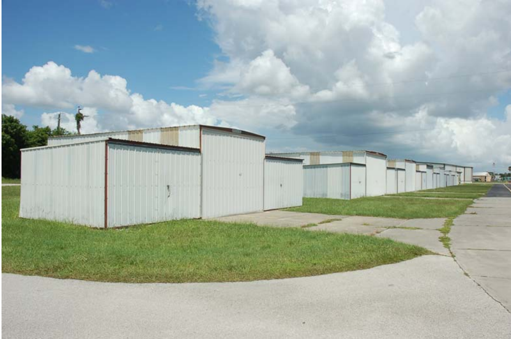
View of the north and east elevations.
