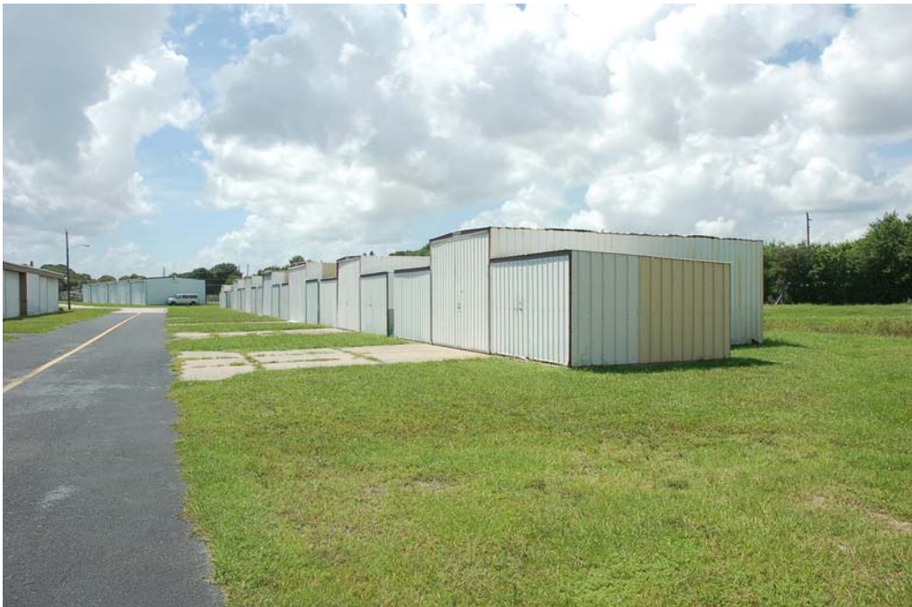
View of the south and west elevations.
