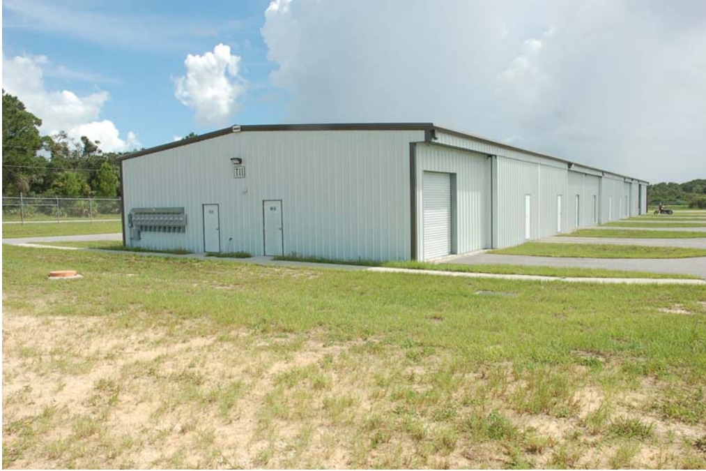
View of the north and west elevations.
