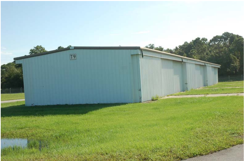
View of the south and west elevations.
