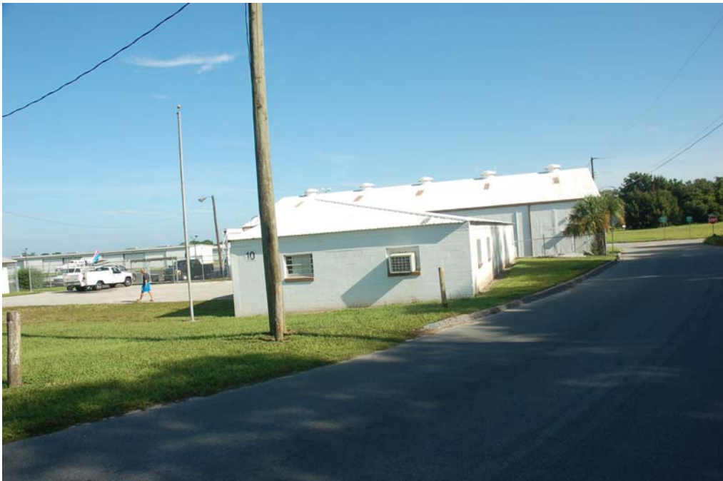
View of the south and east elevations.
