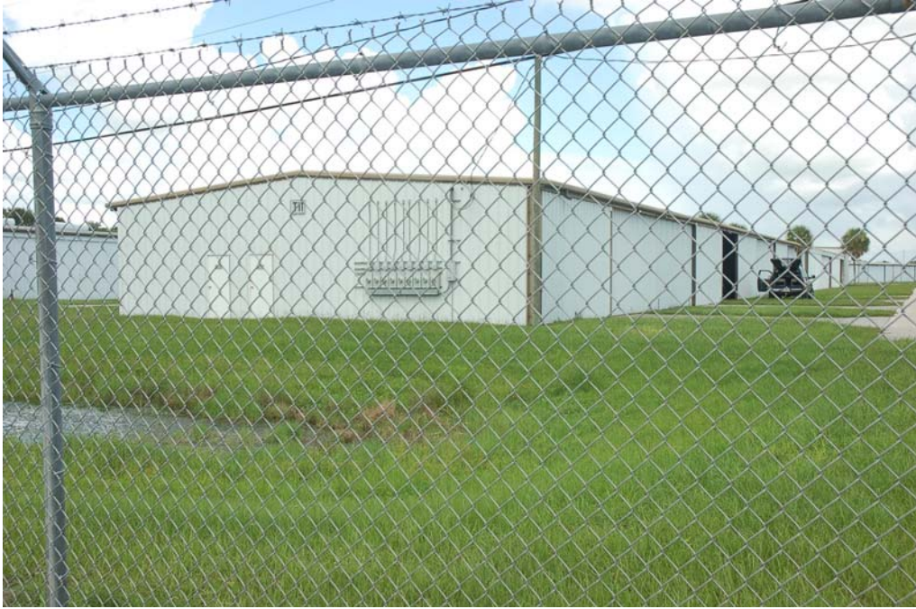
View of the south and east elevations.
