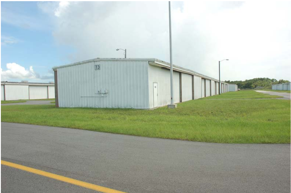
View of the north and west elevations.
