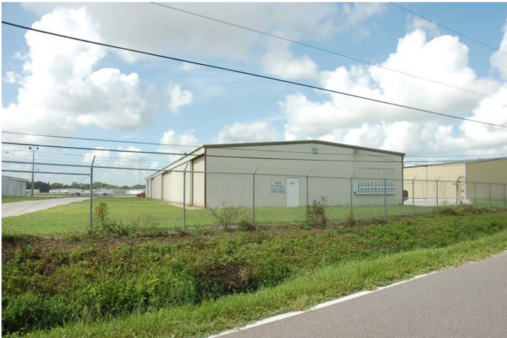
View of the south and west elevations.
