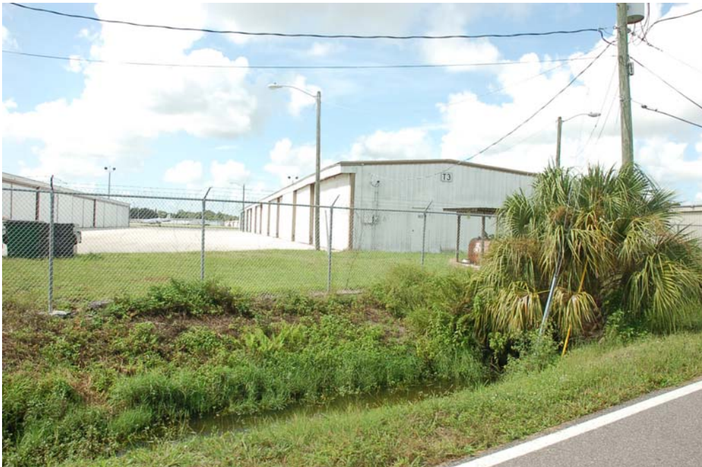
View of the north and east elevations.
