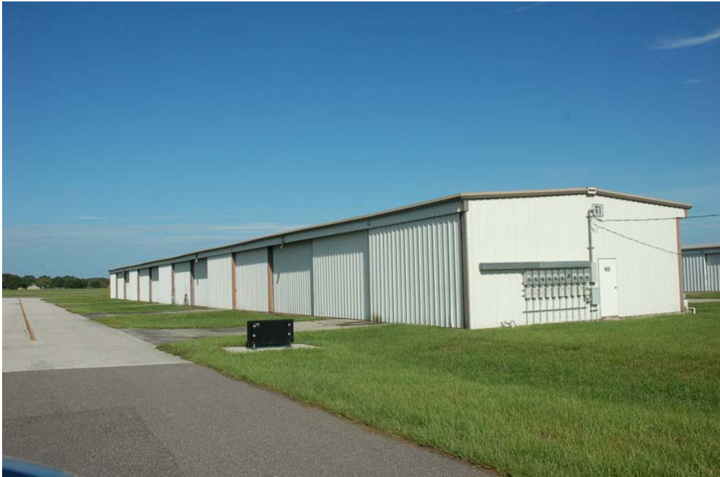
View of the north and east elevations.
