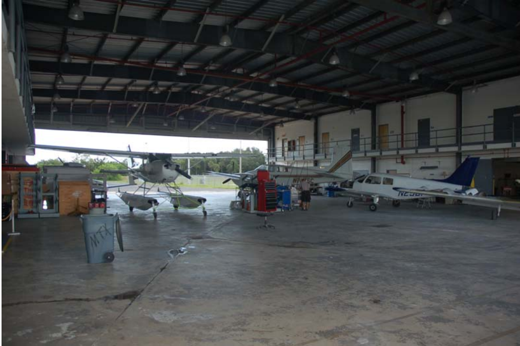
Interior view of hangar area.
