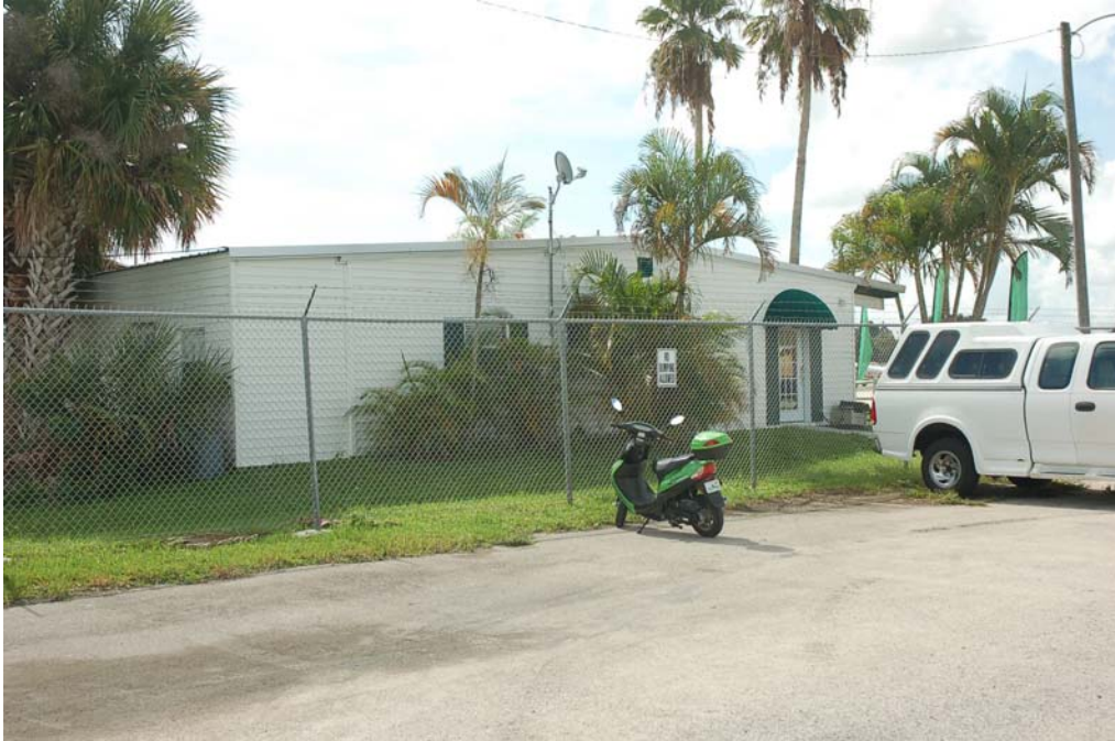
View of the north and west elevations.
