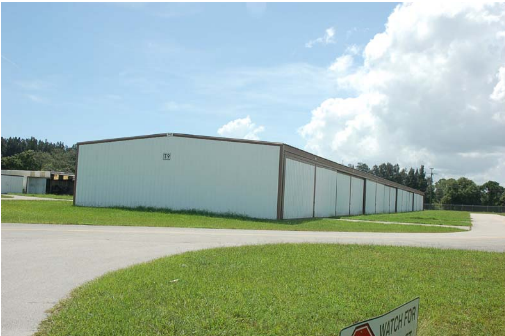
View of the north and west elevations.
