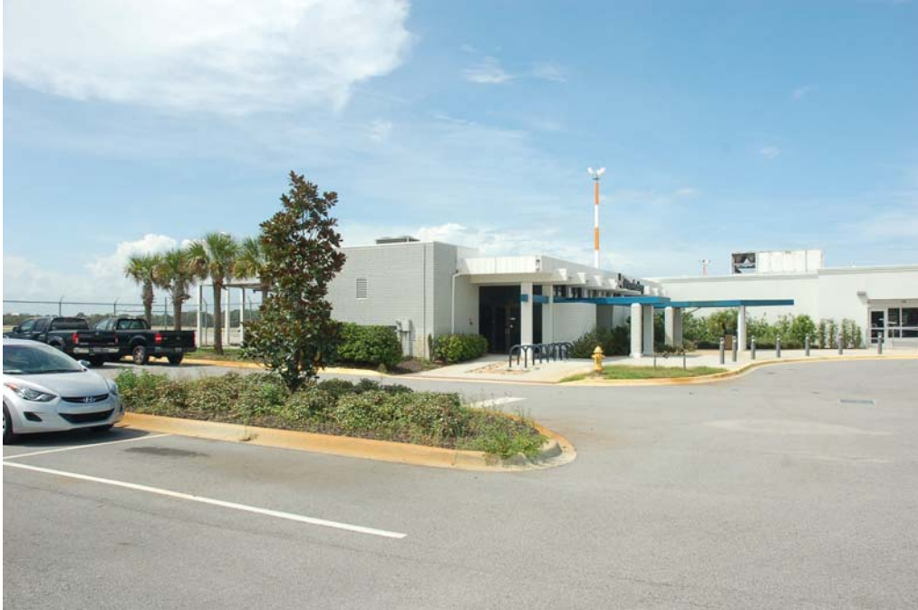
View of the south and east elevations of the original building.
