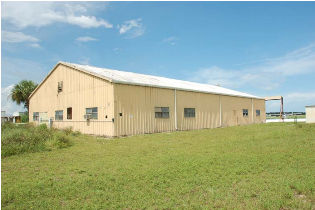
View of the south and east elevations.
