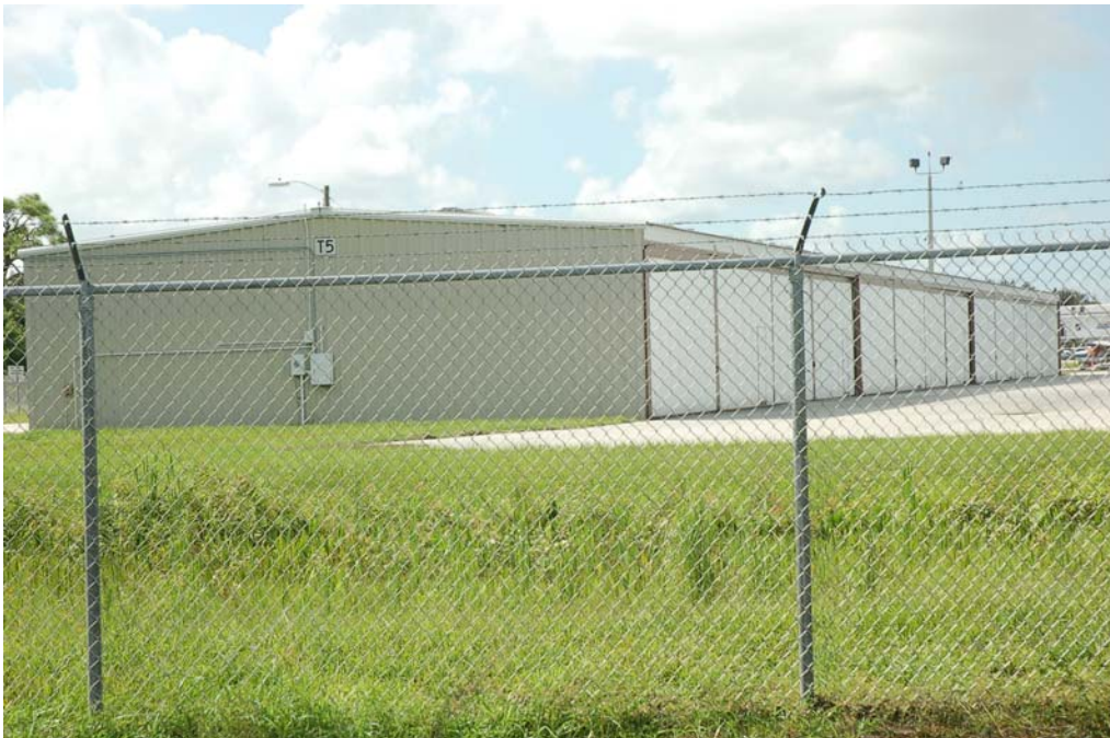
View of the north and west elevations.
