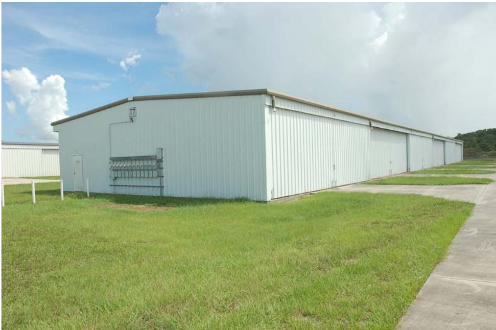
View of the north and west elevations.
