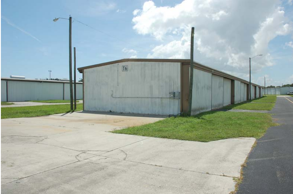
View of the north and west elevations.
