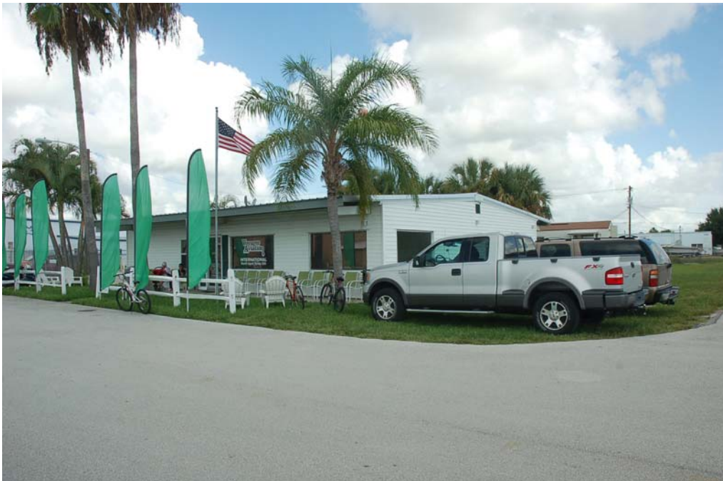
View of the south and east elevations.
