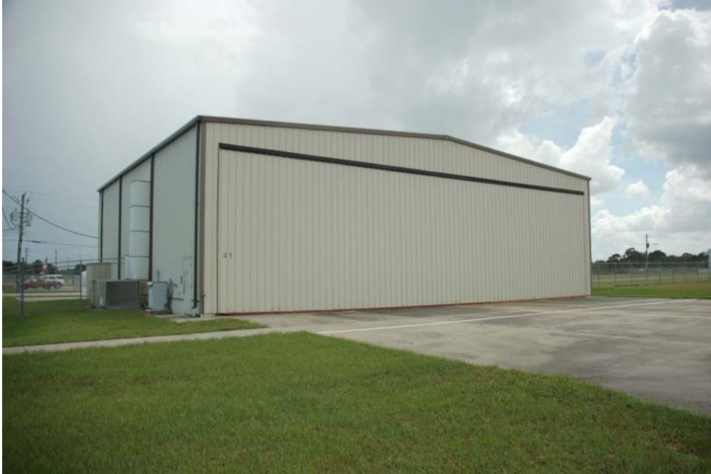
View of the north and west elevations.
