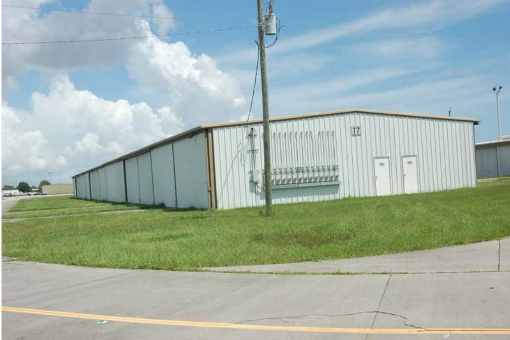
View of the south and west elevations.
