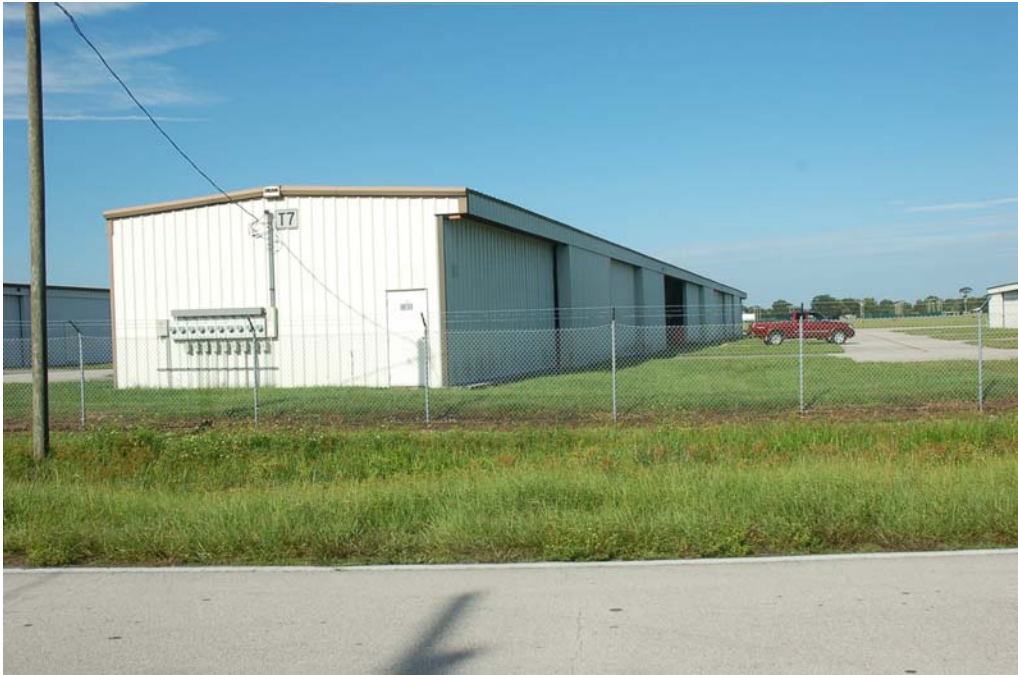
View of the north and east elevations.
