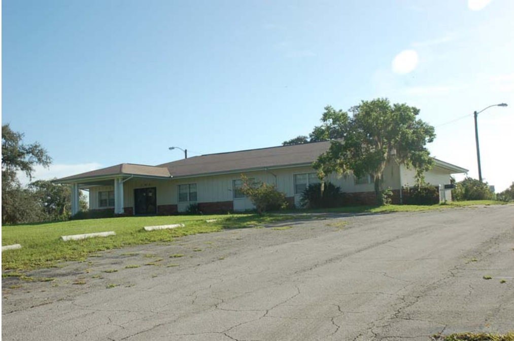
View looking south from Singleton Avenue at the north and west elevations.
