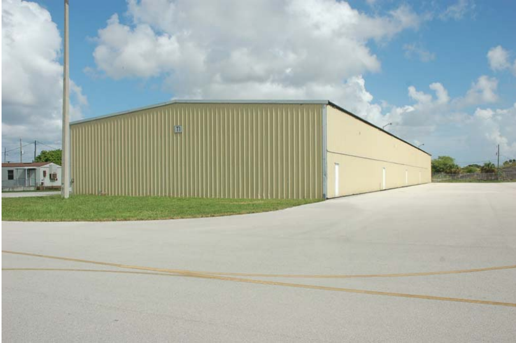
View of the south and east elevations.
