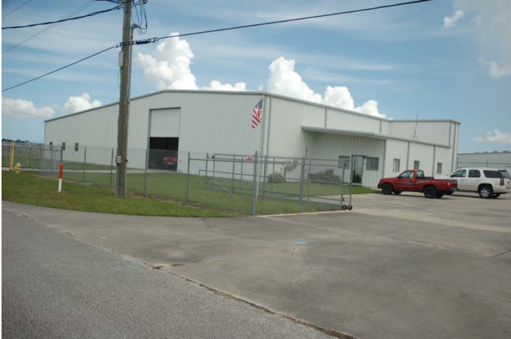
View of the south and west elevations.
