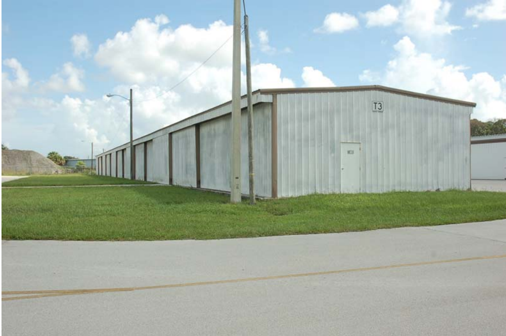
View of the south and west elevations.
