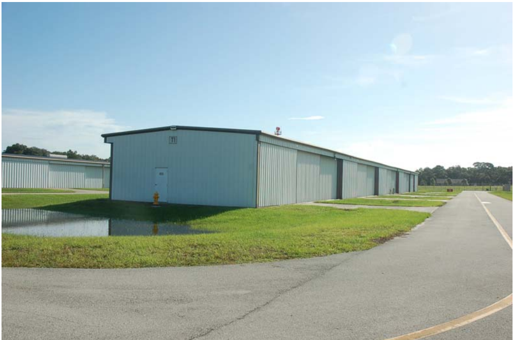
View of the south and west elevations.
