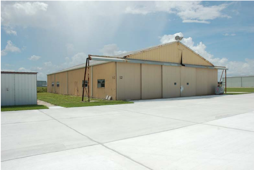
View of the north and west elevations.
