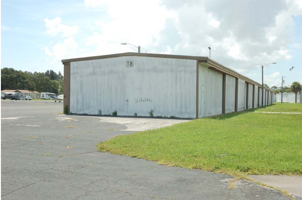
View of the north and west elevations.
