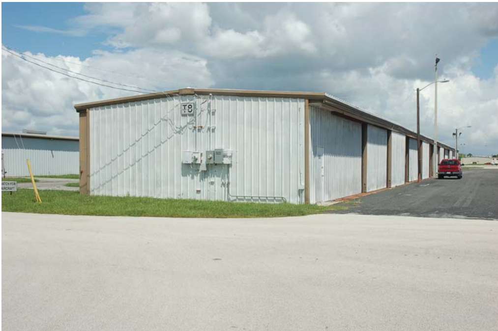
View of the south and east elevations.
