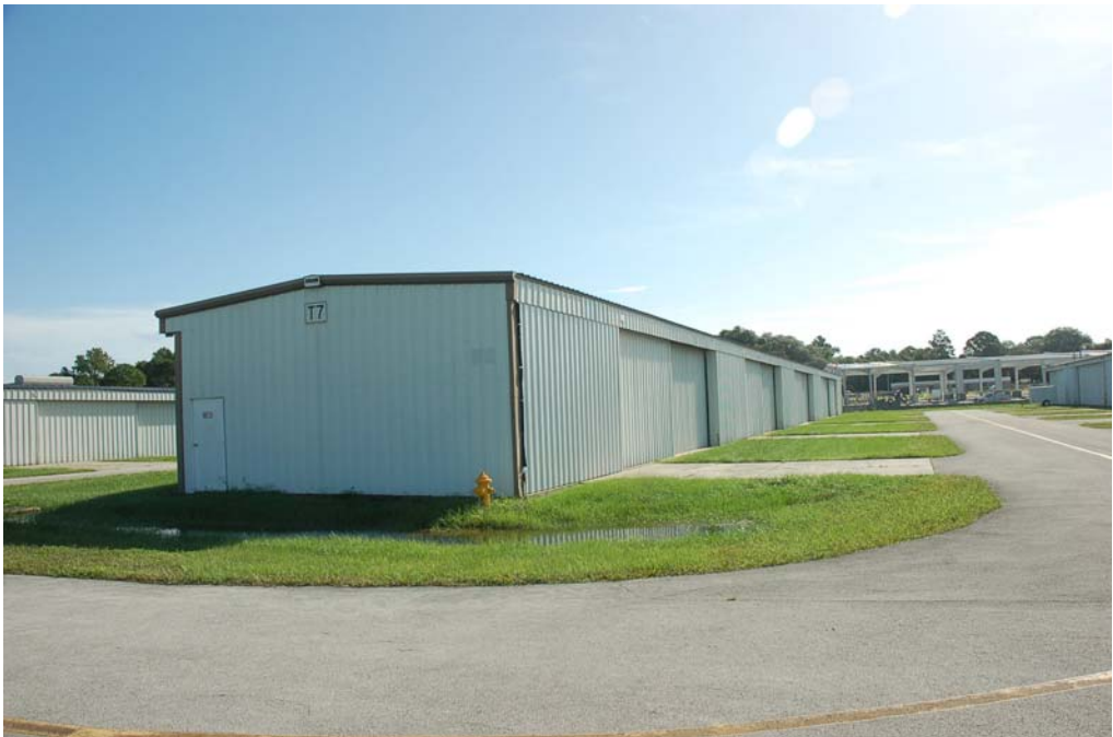
View of the south and west elevations.
