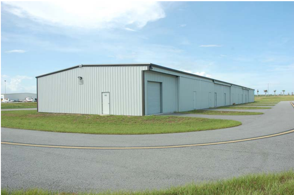
View of the south and east elevations.
