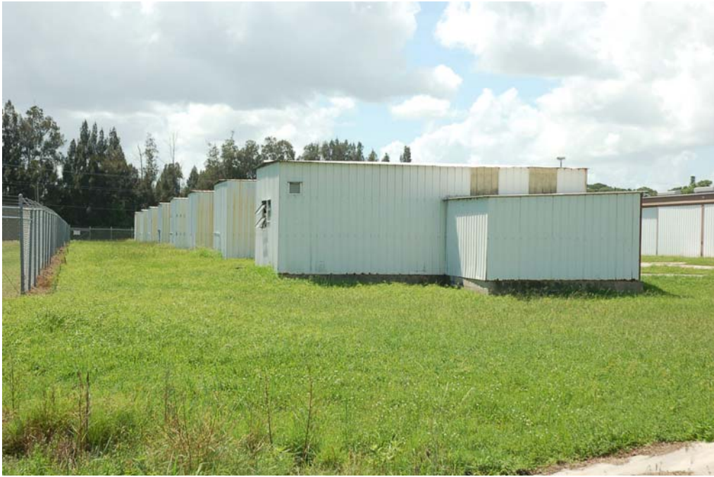
View of the north and west elevations.
