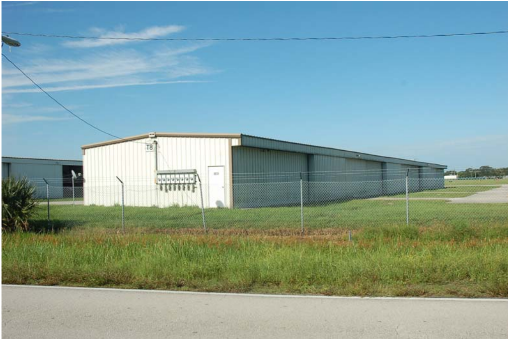
View of the north and east elevations.
