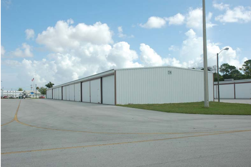
View of the south and west elevations.
