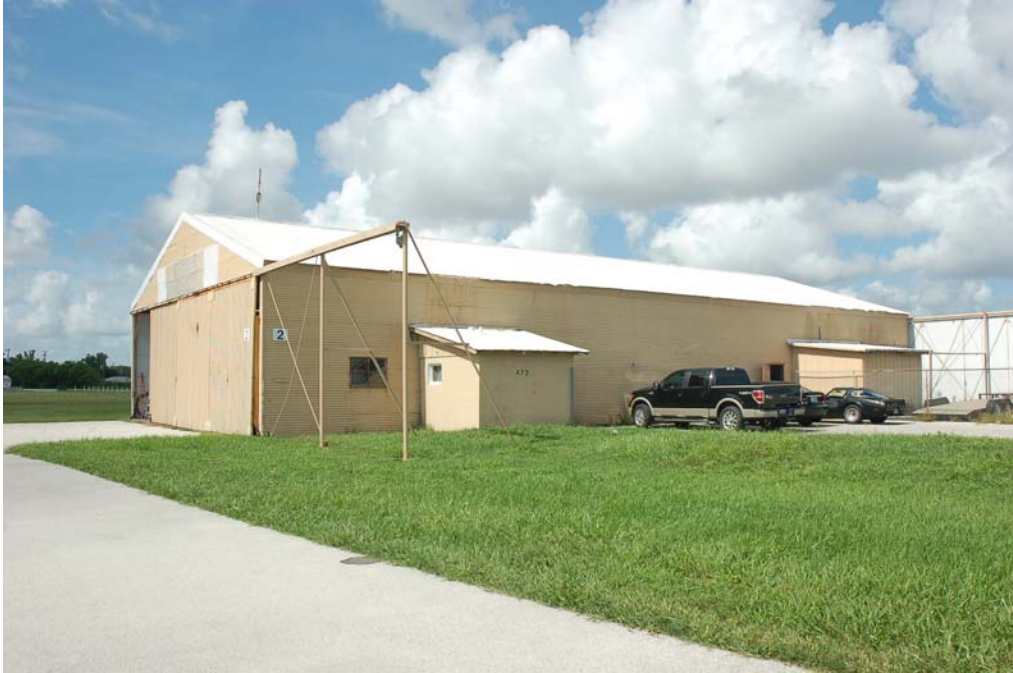
View of the north and east elevations.
