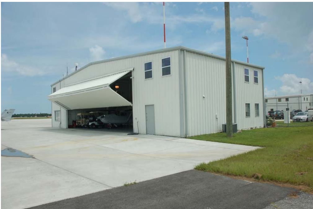
View of the south and west elevations.
