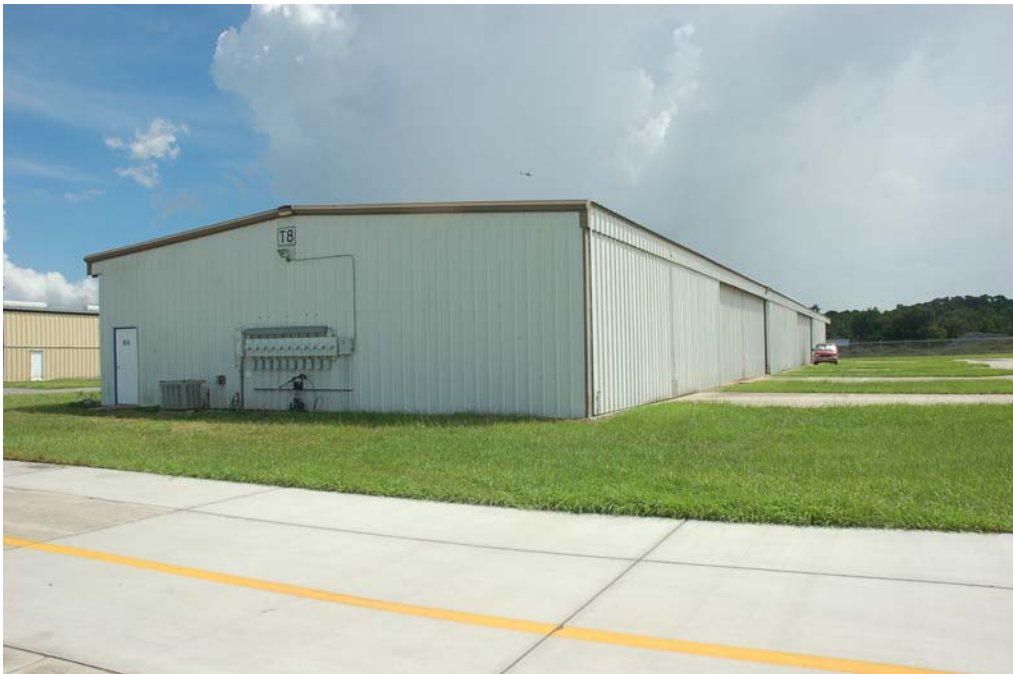
View of the north and west elevations.
