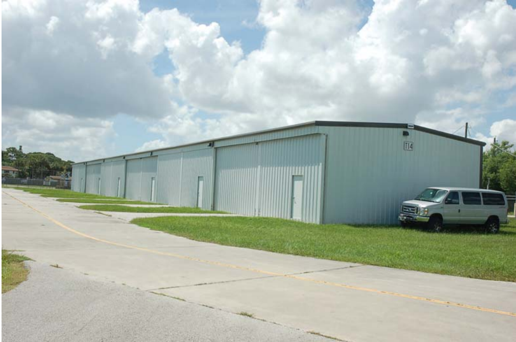
View of the north and east elevations.
