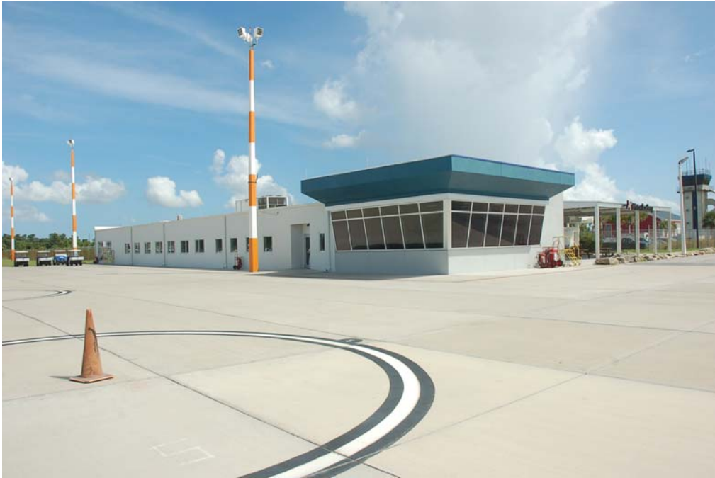
View of the north and west elevations of the new addition.
