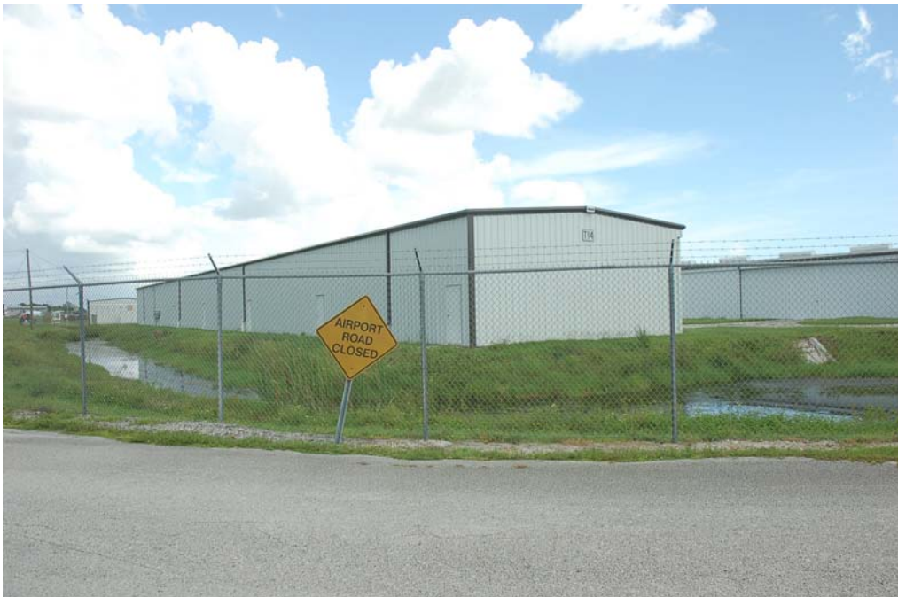
View of the south and west elevations.
