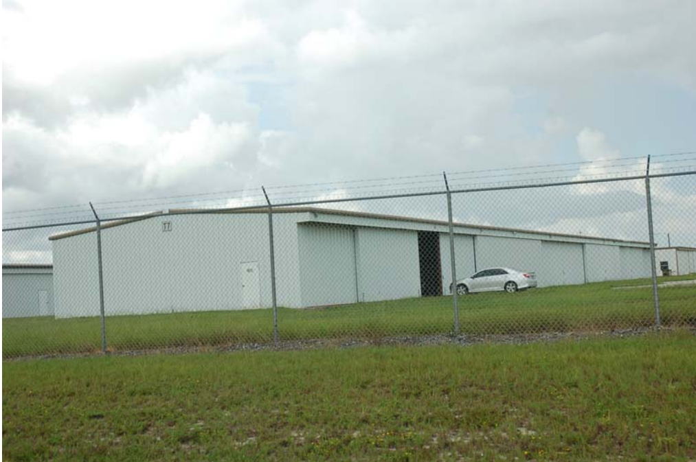
View of the south and east elevations.
