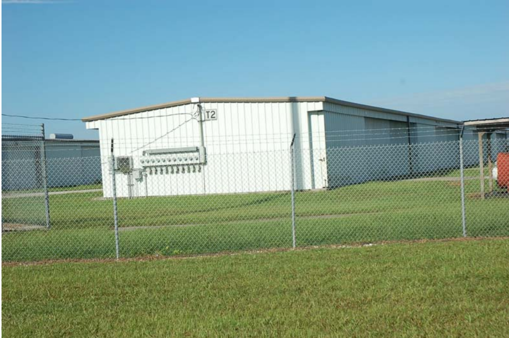
View of the south and west elevations.
