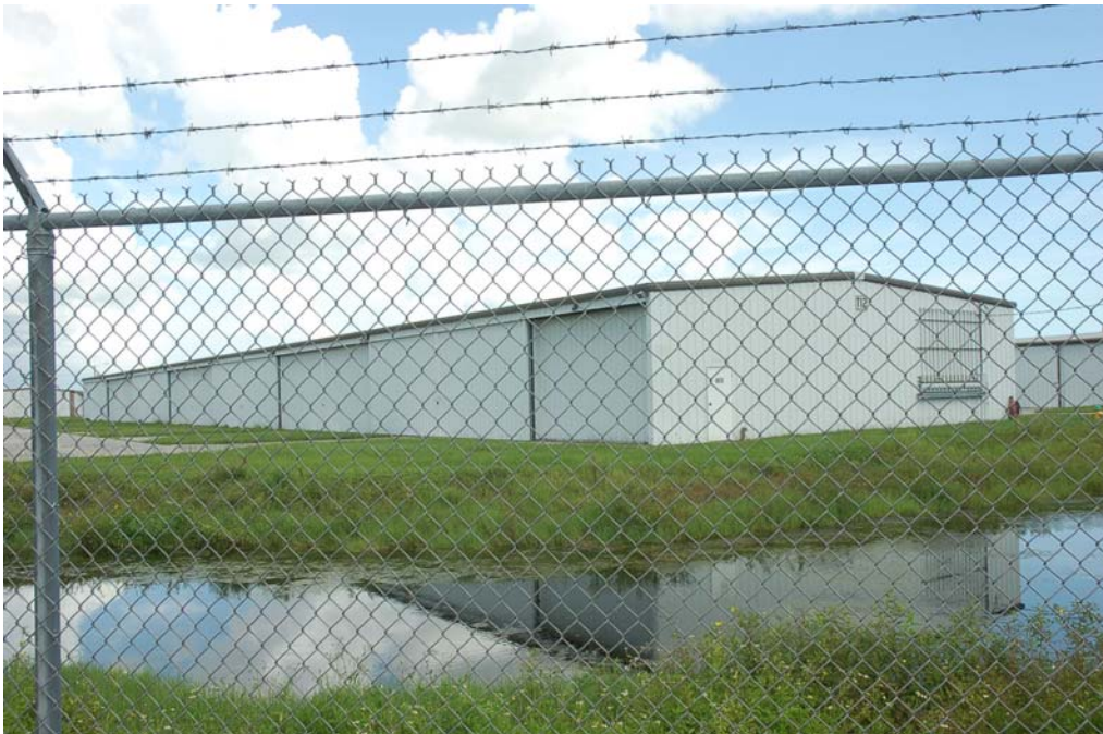
View of the south and west elevations.
