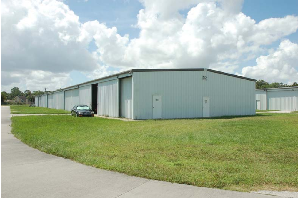
View of the north and east elevations.
