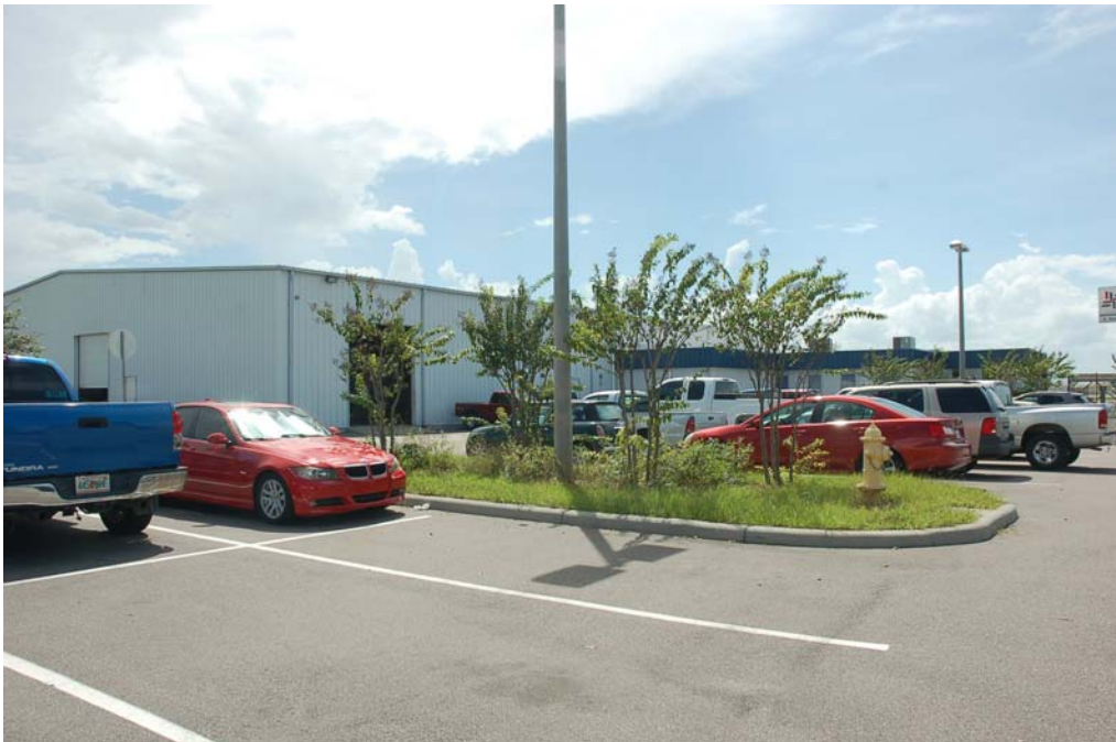
View of the south and east elevations.
