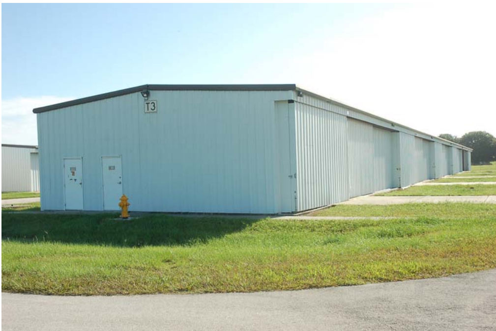
View of the south and west elevations.
