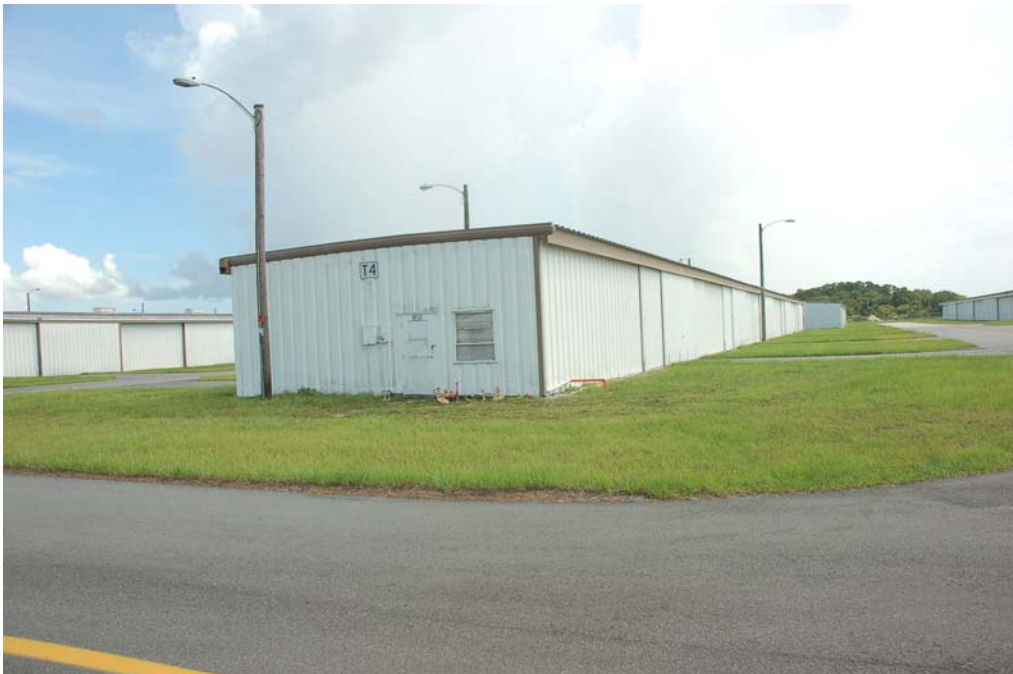
View of the north and west elevations.
