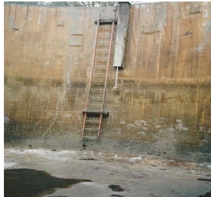
Figure 14: Tank Access Ladder, Int.
