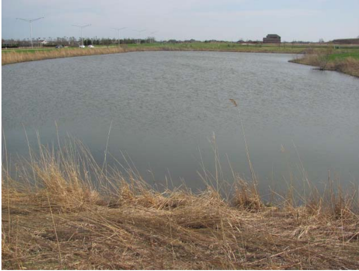
Stormwater Management Area South overview
