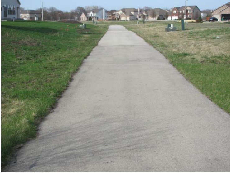
Asphalt walking path west of Portage Lane overview
