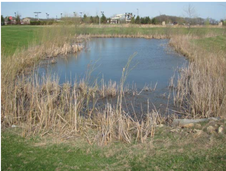
North portion of Stormwater Management Area B
