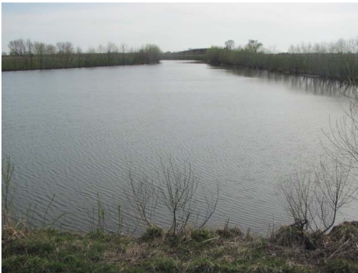
Stormwater Management Area A overview
