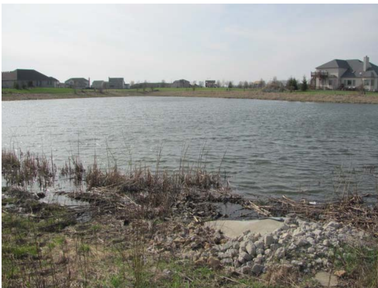
Stormwater Management Area North overview
