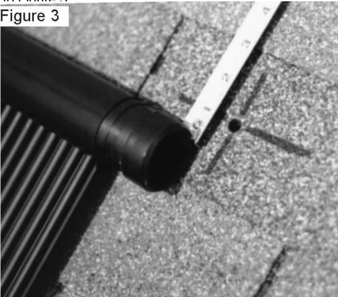
2) Using this point, snap a chalkline to the opposite end of the row. Slope this line down the roof toward the inlet approximately 1" (25mm) for each 6 collectors in the row. Using a 1/8" (3mm) drill bit (for 1/4" (6mm) diameter screws) drill a hole for the first outlet header bracket on the first roof mark. Measure up 1" on center from the first pilot hole and drill pilot hole for second screw. Repeat this process all along the chalkline for the total number of collectors to be installed.
