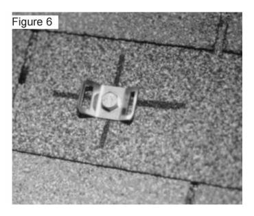
Slip one end of a hold-down strap through the slot in the hold-down strap bracket at the end of the row, then through the strap clamp and out through the other slot in the hold-down bracket. Pull about 3" (7-8cm) of the strap through
