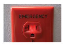
Outlets on the critical-load circuit can be designated for emergency use only. Image: Kristy Johnson
