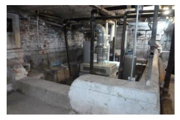
Dry component floodproofing is often an effective solution for equipment that cannot be elevated or relocated out of basements. Image: MAP Architects, New York Engineers.
