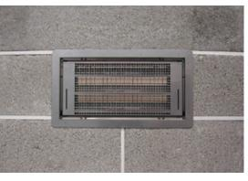
Wet floodproofing vents should be located below the BFE and no more than 1 ft. above the ground. (See Strategy: Elevated Equipment) Image: www.yourfloodrisk.com.
