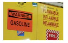
Generator fuel must be carefully stored in code-appropriate enclosures and tanks. Image: Samantha Yost. Develop a maintenance plan that "exercises" the generator regularly and cycles through stored liquid fuel on a defined schedule so you can be sure it will be available and not stale when needed. Train facility staff in equipment operation.
