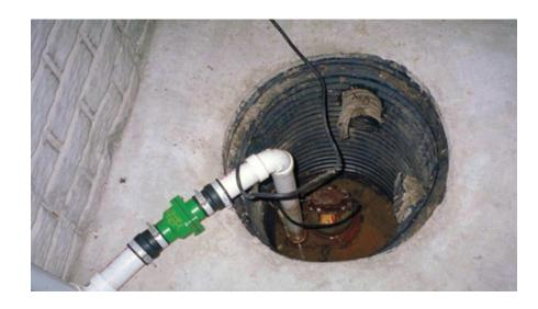
Design sump pumps to handle moderate flooding but not catastrophic flooding such as a coastal storm surge.
