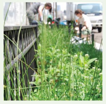
The GCC bioswales are part of a DEP plan to manage stormwater and sewage overflow in the Gowanus sewer shed. Image: Samantha Yost.
