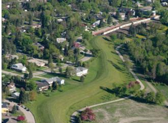
A permanent levee and floodwall system protecting Grand Forks, ND. Image: FEMA / Brenda Riskey
