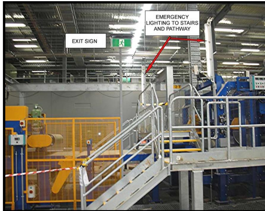
Figure 13 – Local Exit signs and emergency lighting
