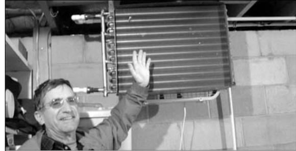
*A solar heating panel feeds this heat exchanger to warm the basement.*
