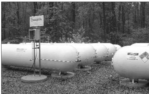
*Hydrogen is stored in low pressure tanks and used to operate a fuel cell during darkness and winter.*
