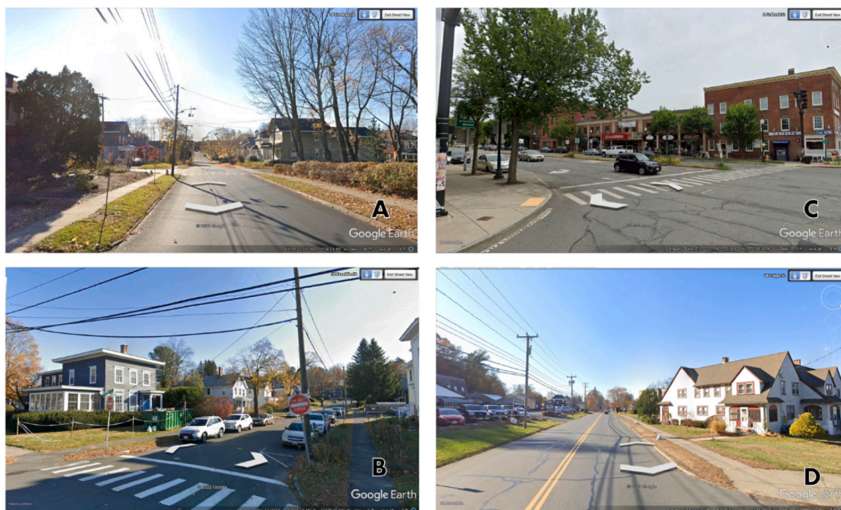
Fig. 4. Examples of typical tree planting space among the built infrastructure of Greenfield, Massachusetts: (A) Residential street with new, small-statured trees planted underneath power lines in the right-of-way; (B) residential street without new trees in the right-of-way; (C) commercial corridor with trees planted in both sidewalk cut-outs and right-of-way planting strip; (D) commercial corridor without trees planted on public or private property (Google Earth, 2022).
