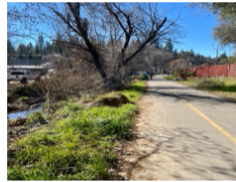
#11 Randolph Creek Project along El Dorado Trail near Hangtown Creek Confluence at Broadway Court
