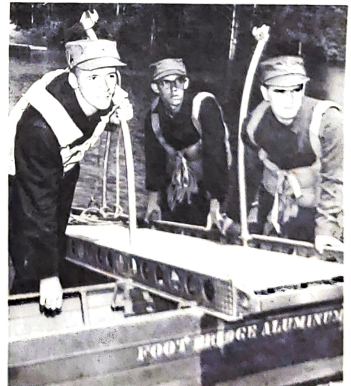
ARMY OFFICER CADETS ON SUMMER TRAINING - O/C's T.W. Coles, left, E.C.M. Bellon, centre, and R. Bunker, right, work on the building and launching of a floating aluminum building at the Royal Canadian School of Infantry, Camp Borden, Ont. They are among 134 Army sponsored first year university students training and training at Army schools across Canada this summer. O/C Coles, a student at McGill University, Montreal, is the son of Mr. and Mrs. William Coles, 113 Pine Beach Blvd., Dorval, Que. O.C. Bellon, a student at Acadia University, Wolfville, N.S., is the son of Mr. Hector W. Bellon, Pine Log Culture, Beauportfield, Que. O.C. Bunker, son of Mr. and Mrs. A.J. Bunker, 150 Michael Rd., Beauportfield, Que., is a student at Royal Military College, Kingston, Ont.
