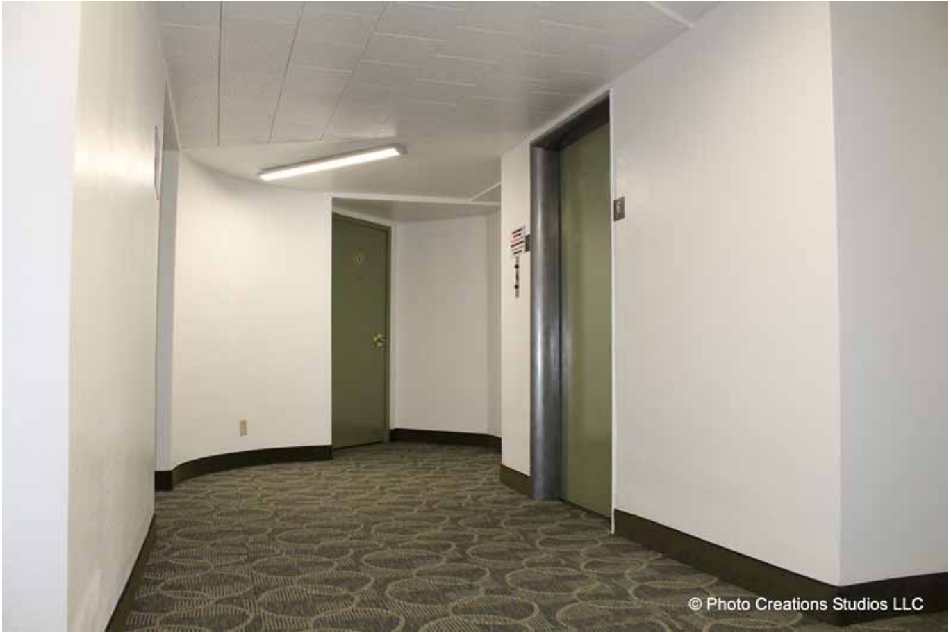
HALLWAY WITH LIGHTING
