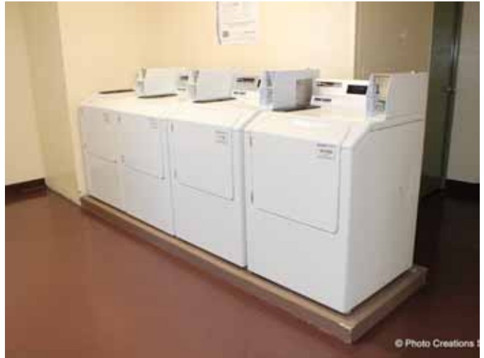
LAUNDRY ROOM – Coin-operated; open 24/7
