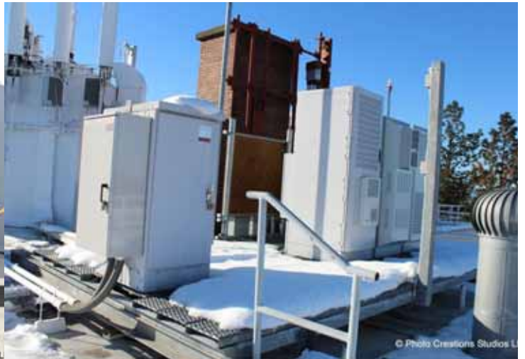
ROOF – CELL TOWER #2
