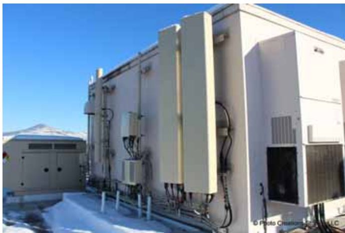
ROOF – CELL TOWER #3
