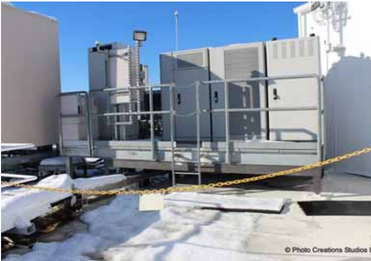
ROOF – CELL TOWER #1
