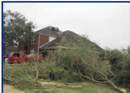
A dislocated chimney on the roof of a house
