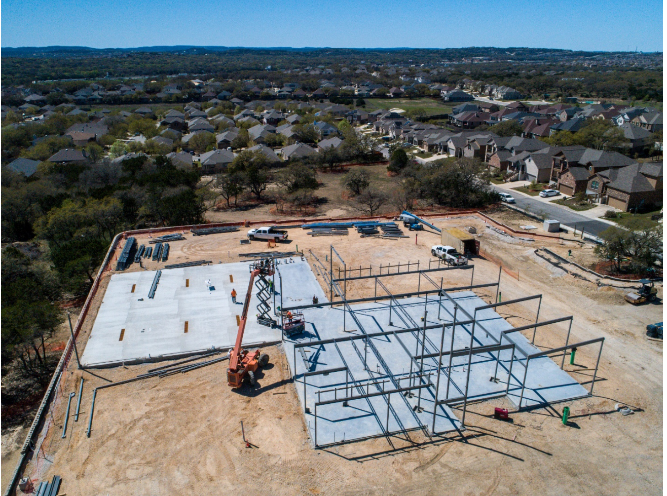
EXHIBIT 1 – FACILITY FOOTPRINT – SLAB & STEEL ERECTION 03.25.21
