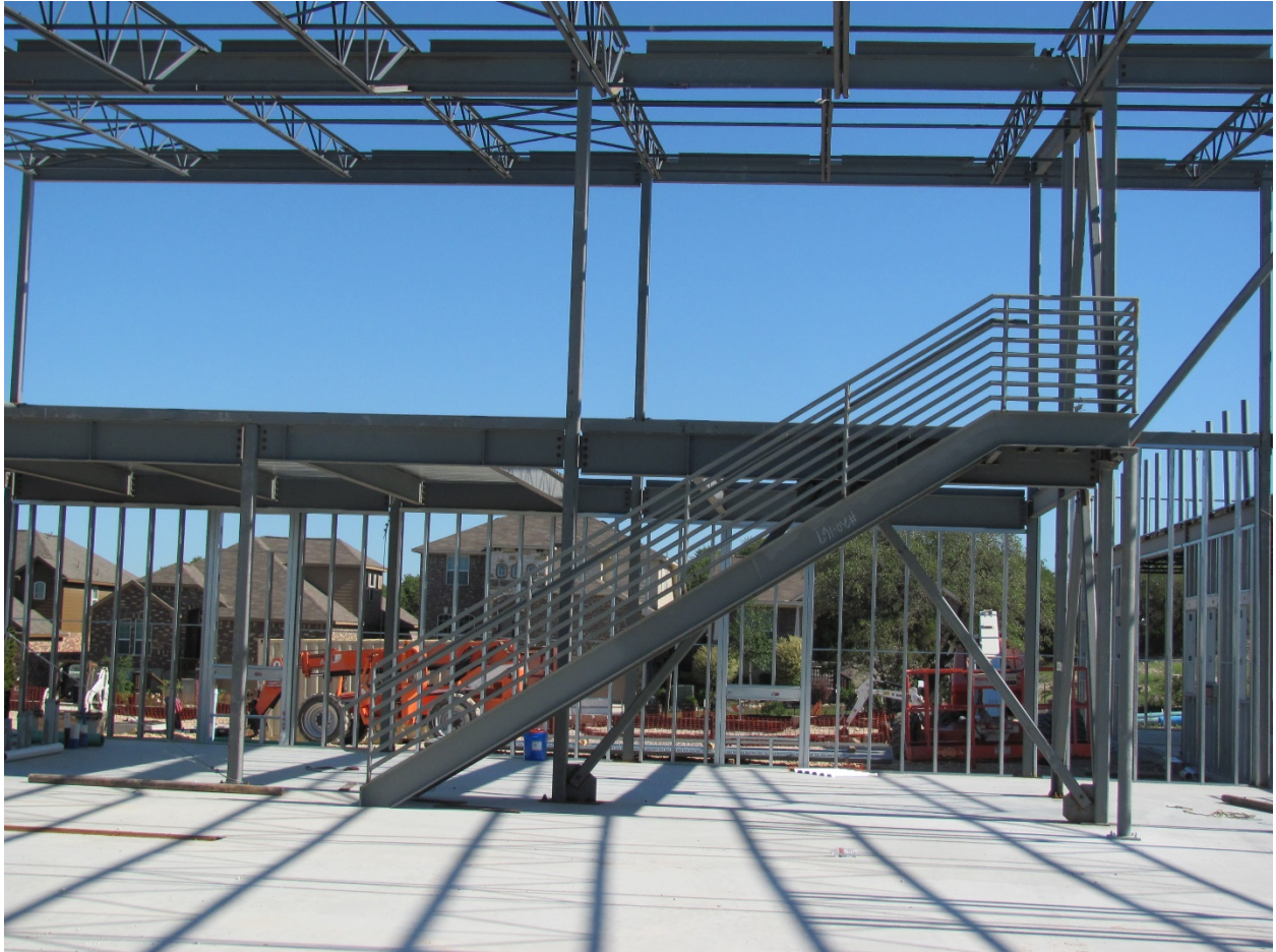
EXHIBIT 4 – STRUCTURAL STEEL – MEZZANINE STAIRS 05.05.21
