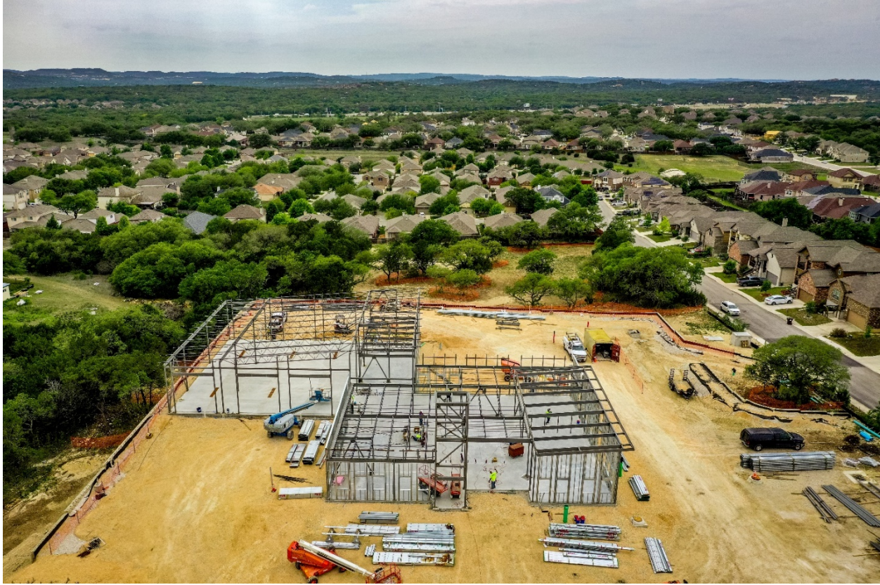
EXHIBIT 2 – STRUCTURAL STEEL ERECTION 04.23.21
