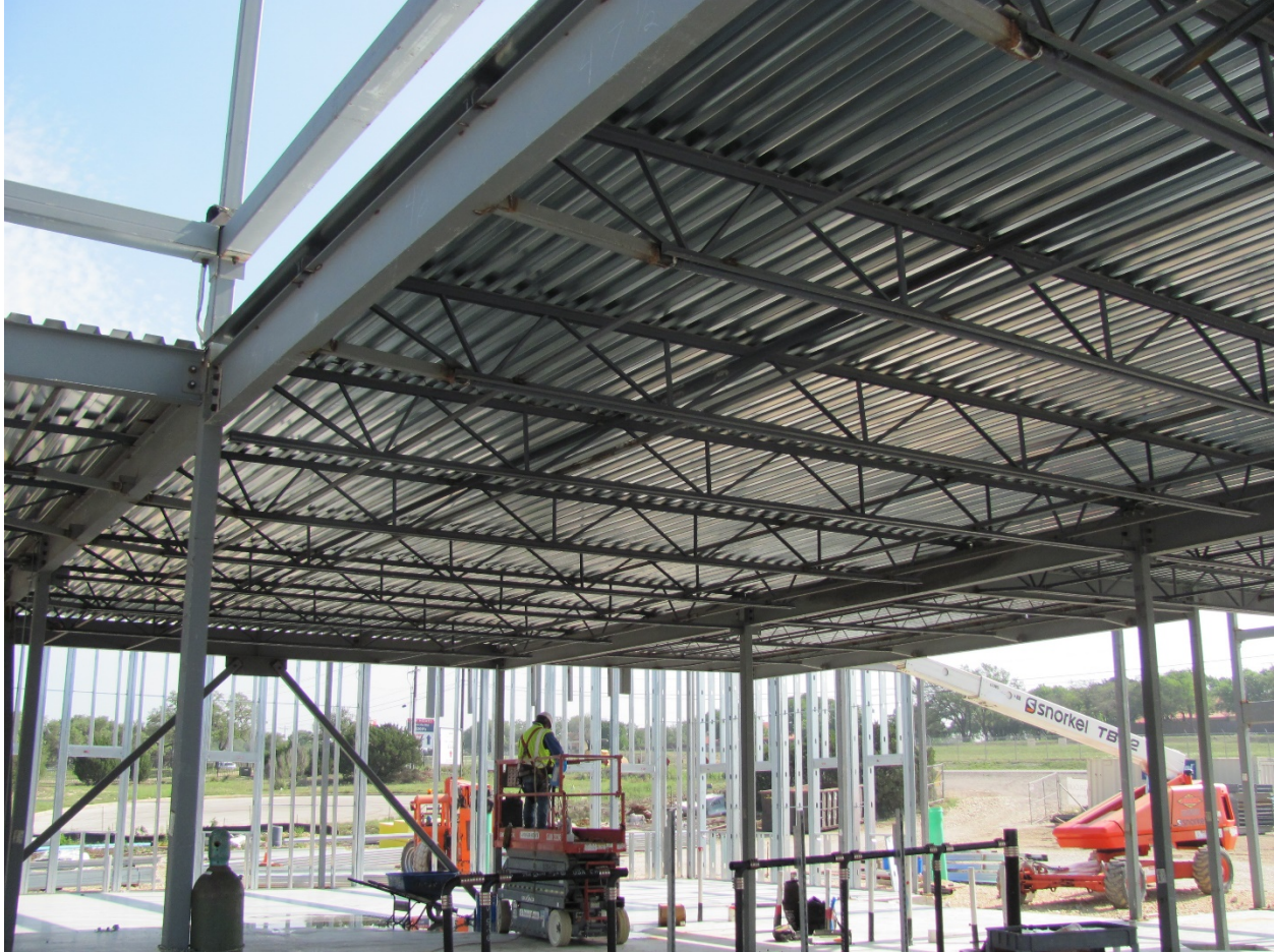
EXHIBIT 3 – ROOF DECKING INSTALL 05.03.21
