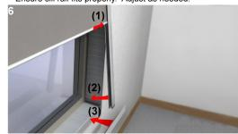
Place hem bar into side channels so hard stops are at top of window opening. Place side channels and sill rail in window opening. Check for plumb and clearance between fabric roll and side channels.
