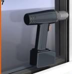
Secure all pieces with screws. Install optional adhesive backed wool pile on sill rail at this time. Position adhesive backed wool pile as needed to block light.
