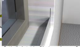
Decide sill rail orientation. Either leg may face room. Predrill sill rail. Position sill rail's outer face flush with window jamb mark. Adjust as needed.
