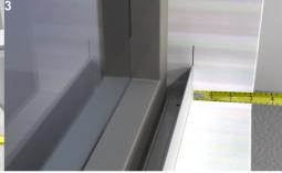
Decide sill rail orientation. Either leg may face room. Position sill rail's outer face flush to window jamb mark. Ensure sill rail fits properly. Adjust as needed.
