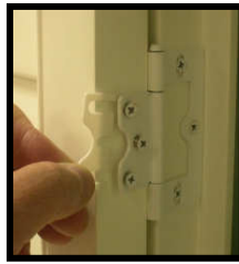
Insert hinge spacer.
