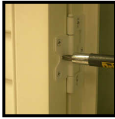
Loosen screws on panel hinge. Do not remove completely.
