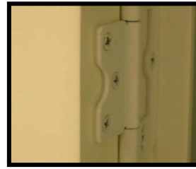
Hinge spacer installed.
