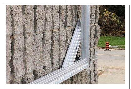
Here the frame was screwed on a piece of TS44 to provide a distance from the rough stone wall
