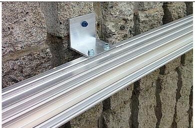
Aluminum brackets were custom made to fix the frame and keep the same distance from the wall.
