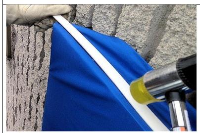
Then the segments are removed and replaced by longer PVC inserts.
