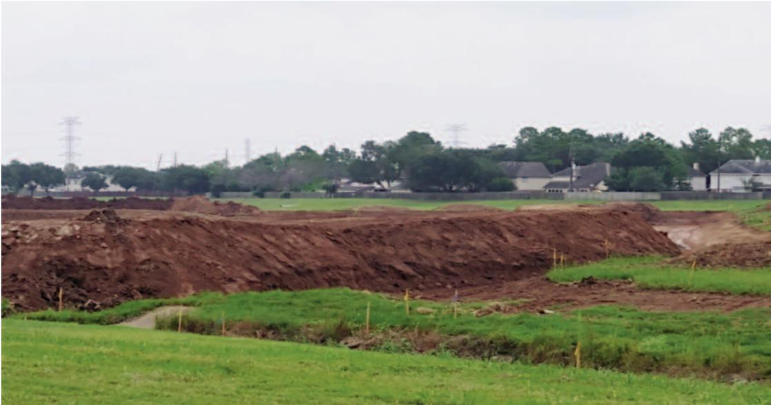
First Colony Levy Improvement District owns the property south of Lexington and west of Brightwater. Currently they have a 60-day project underway to increase the detention capacity of this area. The project entails removing dirt which will be used to bolster surrounding levy systems and in turn will allow more water to be held during heavy rain events. Water flow eventually drains into Oyster Creek. The land will be hydro-seeded after construction.
