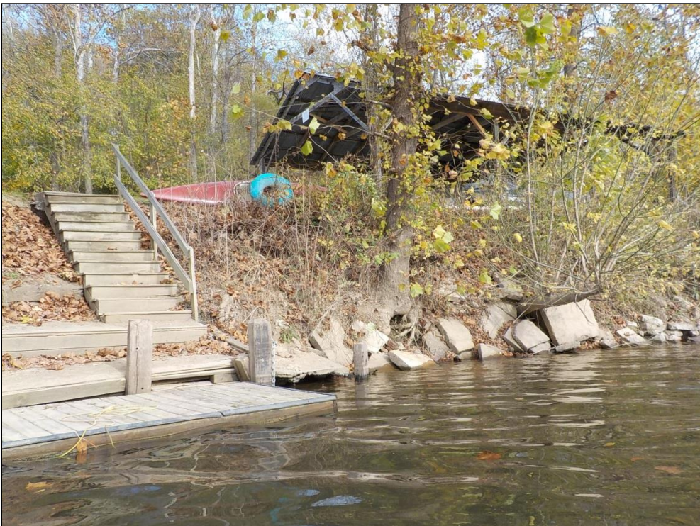
Photograph 14 – Typical NE riverbank land use/development (note rock/riprap), view N
