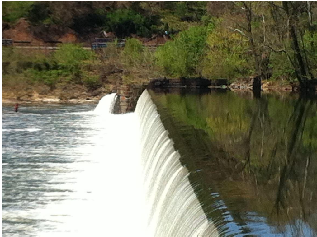
Photo 7 – Scott's Mill Dam April 2016 – 1,800 cfs
