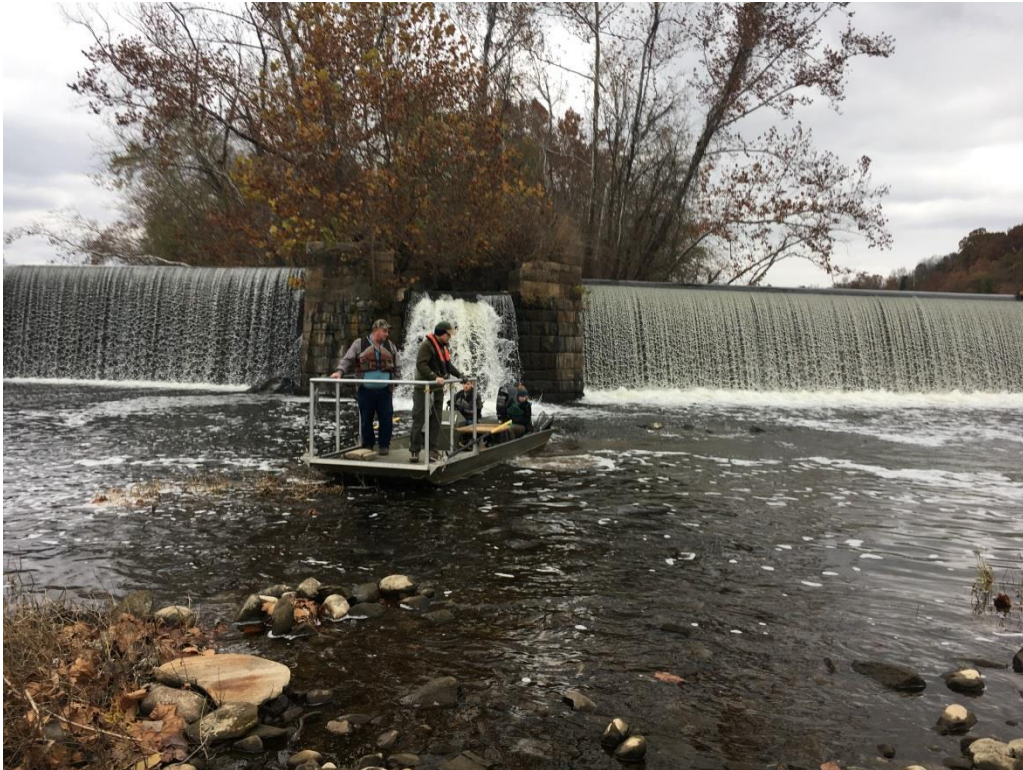
Photo 9 – Scott's Mill Dam November 14, 2017 – Flow 1,500 cfs – Note Flow Over Arch Section and Old Fishway
