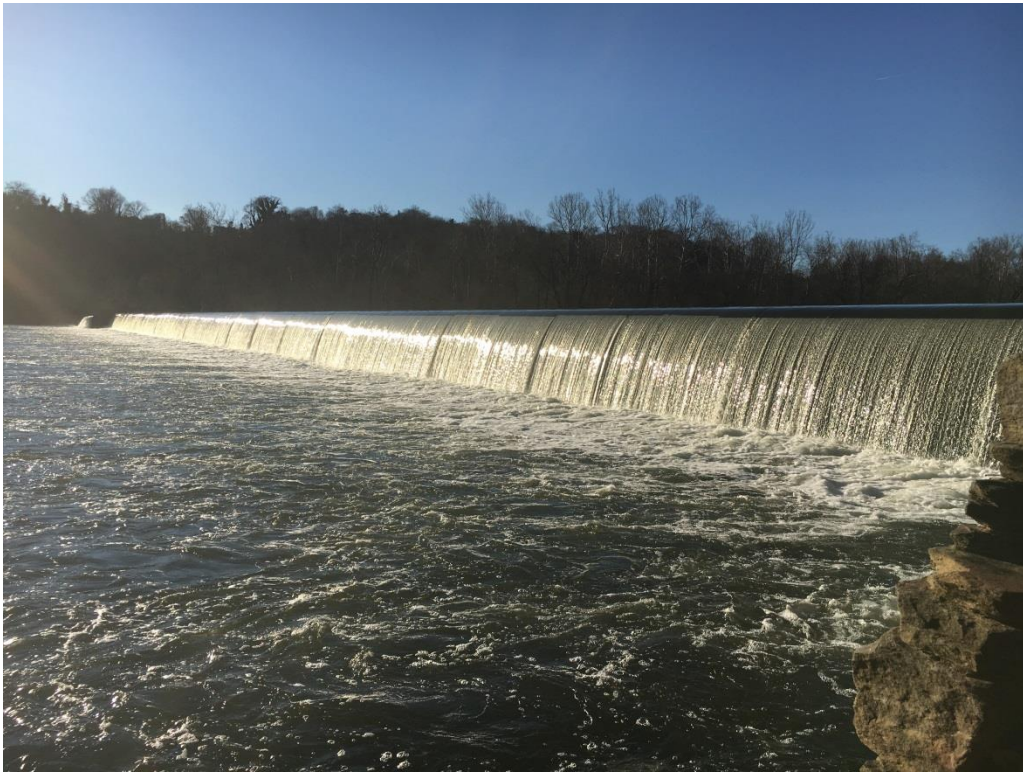
Photo 13 – Scott’s Mill Dam February 2, 2017 – Average Flow 3,200 cfs
