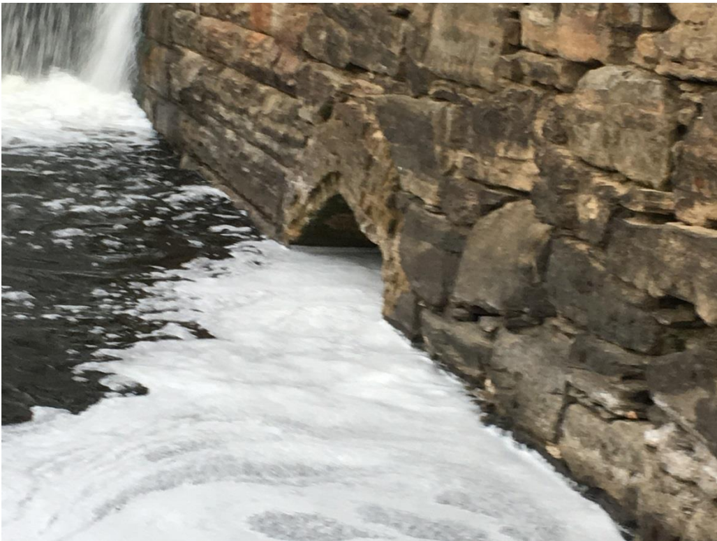
Photo 23 – November 28, 2016 View of Scott’s Mill Grist Foundation (Left Abutment) Showing Grist Mill Discharge Location
