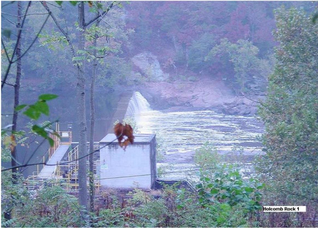
Photo 5 – Holcomb Rock Dam
