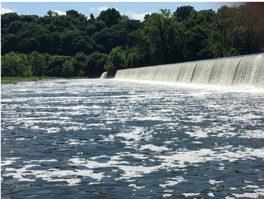
Photo 12 – Scott’s Mill Dam July 7, 2017 – Flow 1,400 cfs
