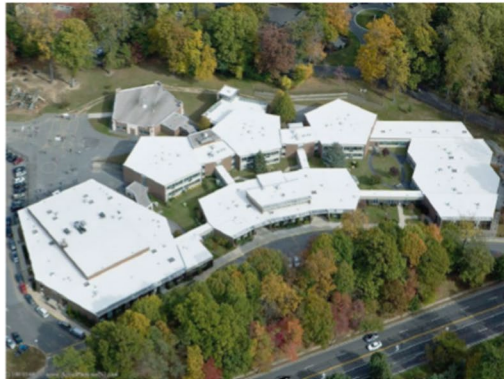
Low-slope roofing membrane installed using low-VOC adhesive and consisting of a SBS-modified bitumen cap sheet and base sheet.
