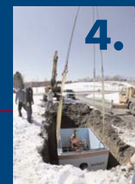
Vault base positioned on site 11:20 am
