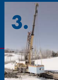
Vault base unloaded 11:15 am
