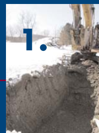
Initial site prep
