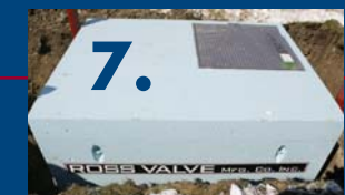
Vault ready for connection 11:55 am
