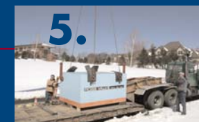
Vault top unloaded 11:30 am
