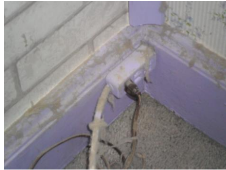
Remove extension cord wiring
