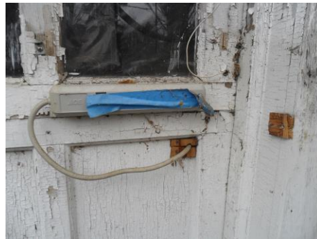
Improper exterior electrical
