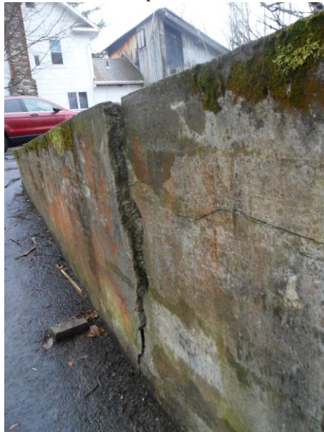
Cracked and leaning retaining wall into basement
