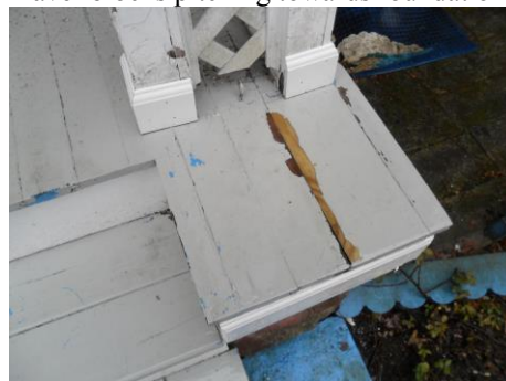
Peeling paint on front porch deck
