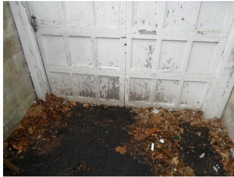
Bare wood exposed on basement entrance
