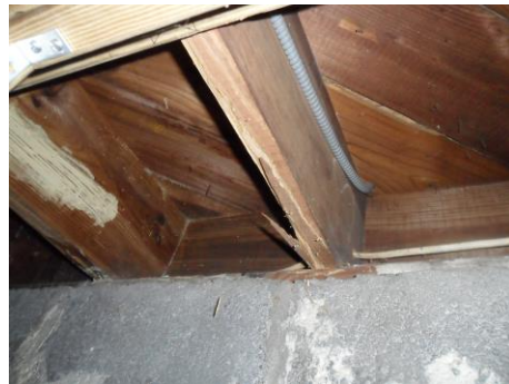
Monitor evidence of old terminate damage
