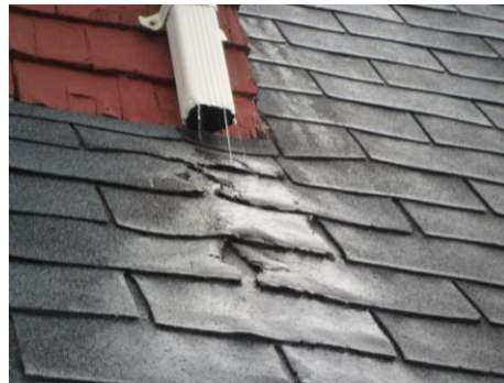
Damaged roofing shingles
