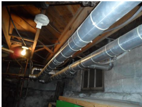
Evidence of asbestos wrapped piping
