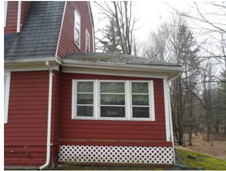
Monitor excessive pitch on side porch
