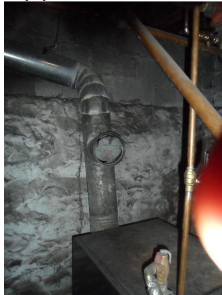
Evidence of soot back up recommend cleaning
