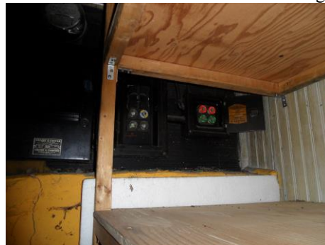
Recommend service upgrade to breakers
