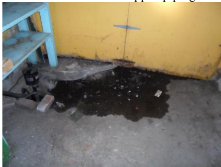
Water seepage recommend directing to pit
