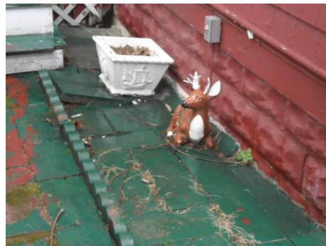
Paver blocks pitching towards foundation
