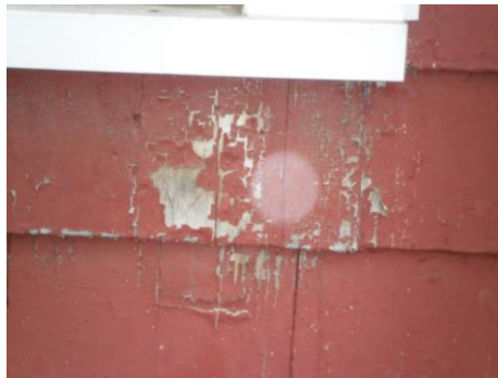
Peeling paint on cedar siding
