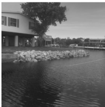
Rip Rap Seawall
