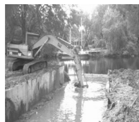
We do Dredging
