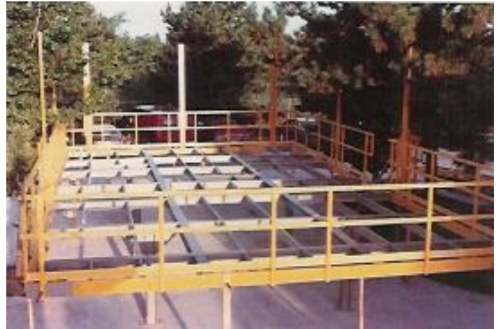
Preassembly of well bay platform of Glass-Steel plant.
