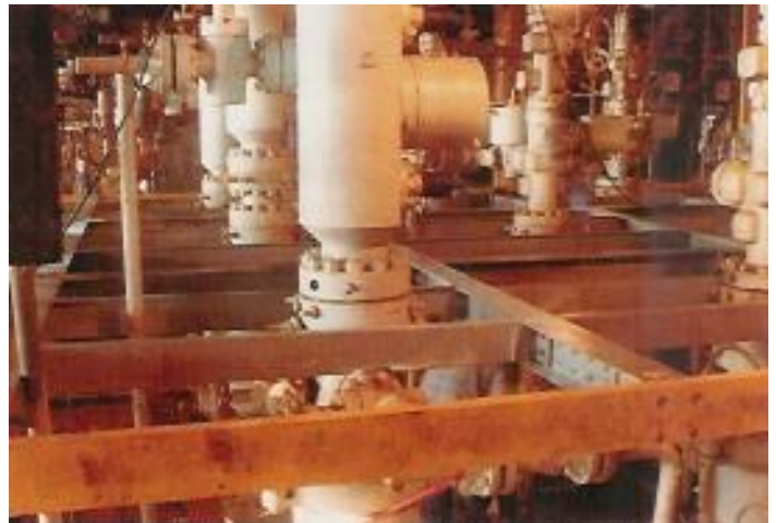
Final assembly of platform in progress on Southpass 62.
