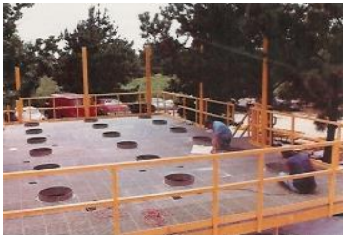
Grating with well holes are added to preassembly.
