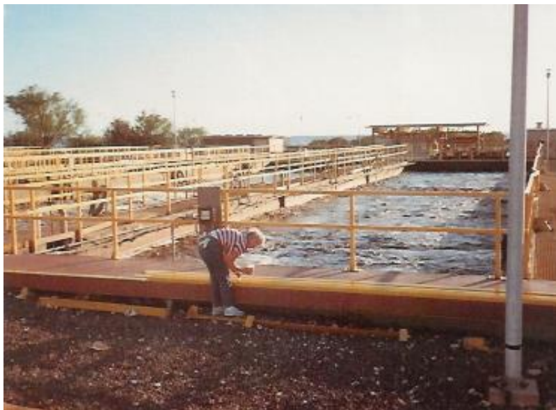
2500 feet of Glass-Steel handrail was installed in 1984 at the Fort Kamehameha Wastewater Treatment Facility, Pearl Harbor Naval Base in Hawaii.
