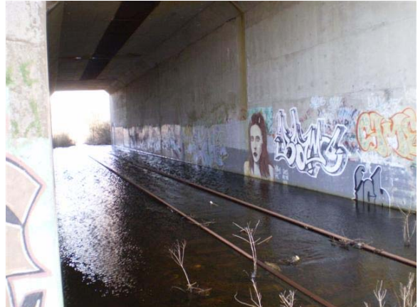
Figure 5: Saugus River Overflow Towards Wakefield Under the Route 95/128 Bridge
