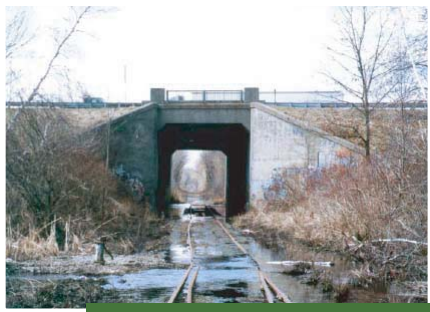
Route 1-95 Bridge over rail trail.
