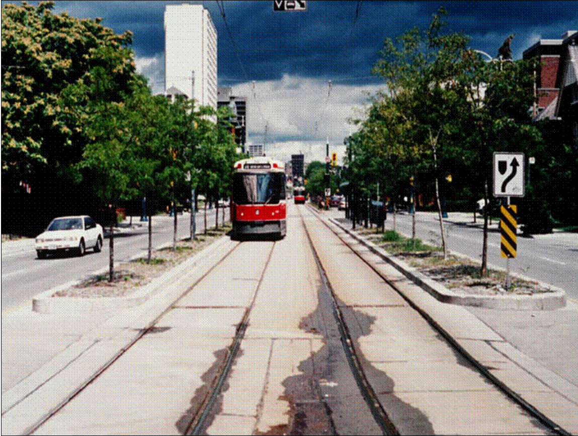
Median streetcar right of way along Spadina Avenue in Toronto (note the landscaped curbing that protects exclusive portions of the right of way) – photo courtesy IBI Group, Inc.
