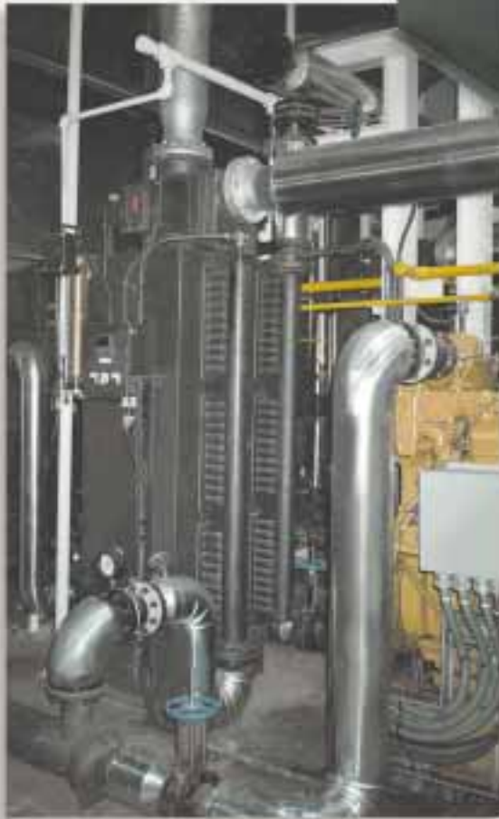
HOSPITAL, Ontario (2) Model HRSR-336B28CSS Recovering Btu from (2) Cummins Wäertsilä CW180, natural gas engines. Reducing each 968°F @ 3,666 SCFM to 339°F. Raising 175 GPM hot water from 195°F to 229°F.
