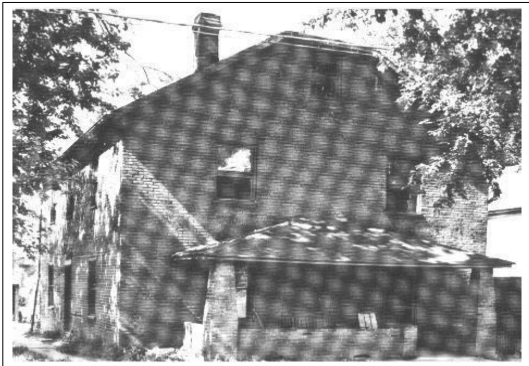
The Buck Inn, built in 1837 at Delmar and State Street.
