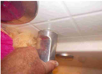
Tub spout is not sealed and could allow water to penetrate behind the tub enclosure
