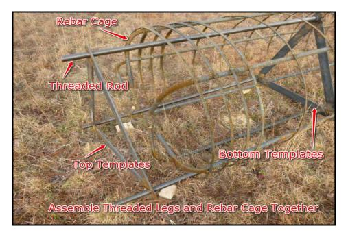
When you do have the legs and cage lowered into the ground, position the three legs so that the tower will be able to hinge over in the desired direction for that installation. Tower will 'hinge' over on one of the three 'sides' of the triangle when base is completed.
