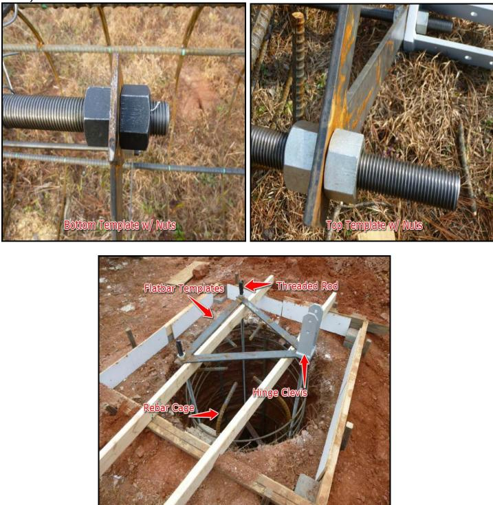
When attaching the steel "U"-shaped welded clevises to the threaded ground bolts, make sure they will be rotated so that all three are in parallel alignment. This will allow the tower to be hinged over for easy erection and section assembly. Small towers may be walked up by one or two persons.
