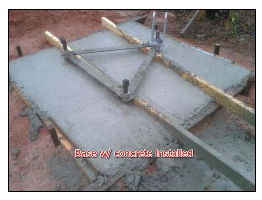
*Curing:* Allow concrete to set for at least 7 to 10 days before installing the complete tower.
