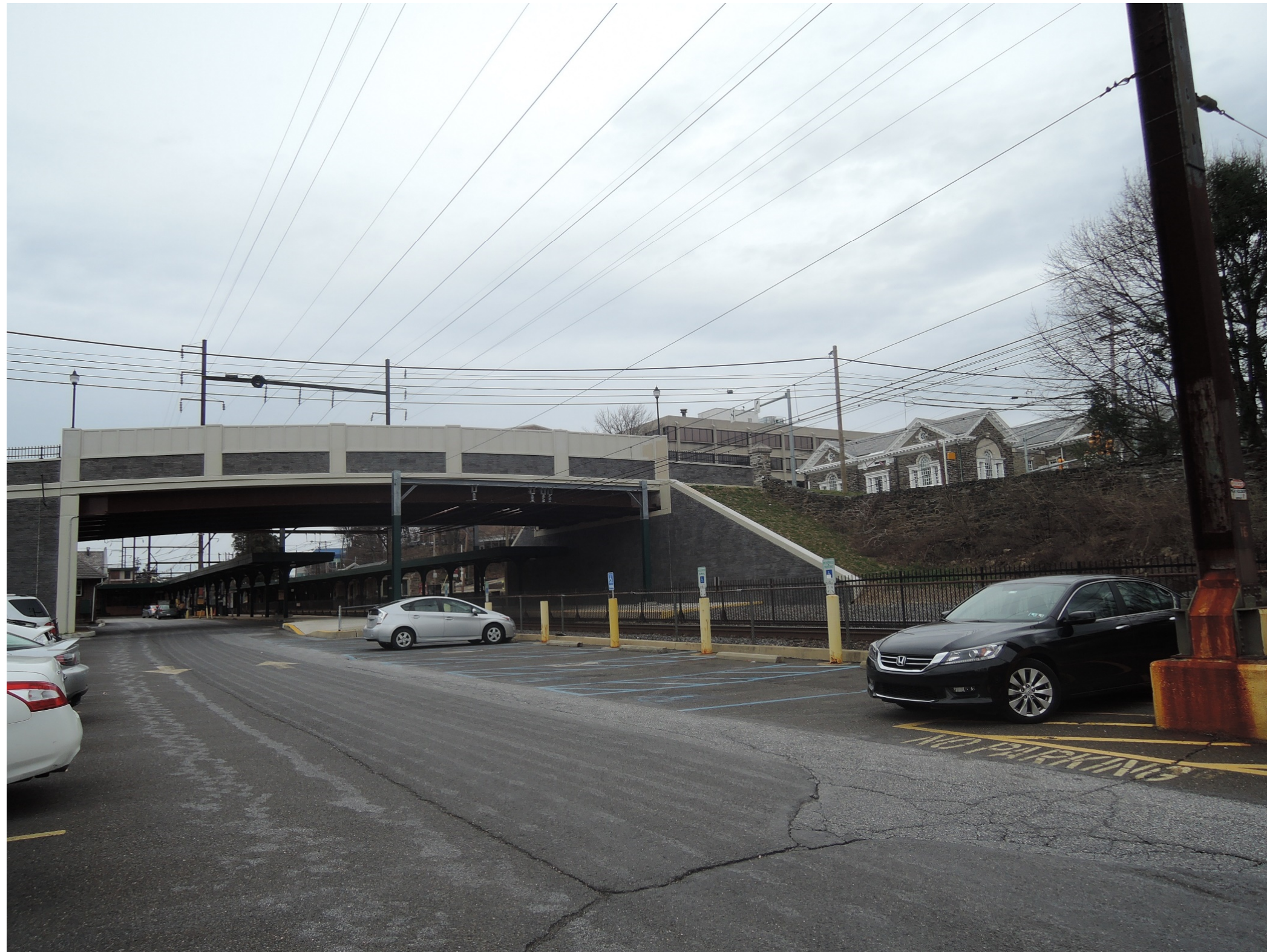
Figure A2 View of Existing Greenwood Avenue Bridge Looking North
