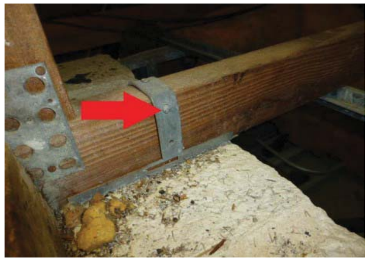
#4 ROOF TO WALL ATTACHMENT OPPOSITE SIDE
