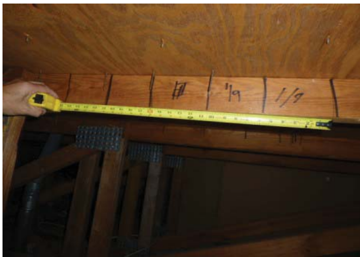
#3 ROOF DECK ATTACHMENT
