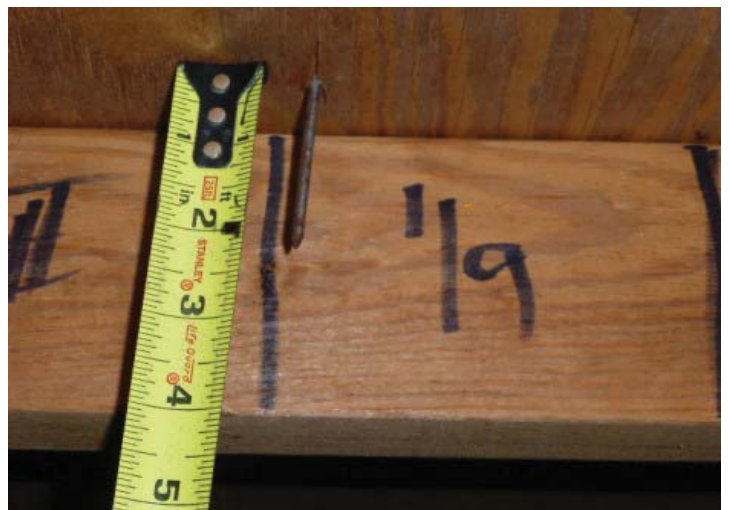
#3 ROOF DECK ATTACHMENT
