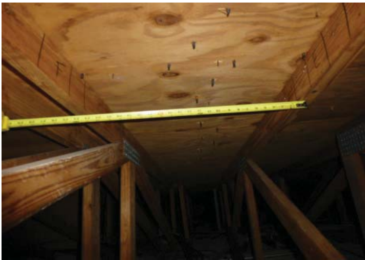
TRUSS/RAFTER SPACING
