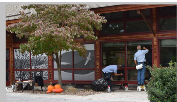
Installation of the CollidEscape on the front of Shuster Hall. Photo courtesy of Jess Murray.
