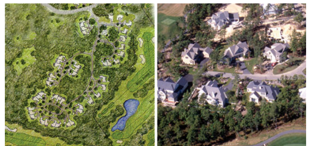
Individual Lots May Be Reduced In Size To Provide For Common Site Amenities Such As Walking Paths, Recreation Facilities and Natural Spaces.
