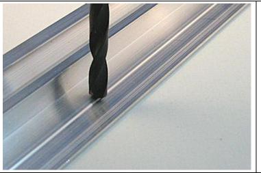
Same process as non-moving vehicles. After having measured, miter the corners, cut the TS23 extrusions to the desired length, you are ready to fix the frame. Start screwing the extrusions to the truck , or trailer sides (one metal screw every 12") You will get a solid frame to install your graphic.
