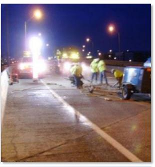
DMTPILNL The PIL NiteLite can illuminate approximately 700 sq. yds./ 64000 sq. ft. it is lightweight and portable. It can be easily stored in the trunk of a car. It takes 15 seconds to inflate and 3 minutes to fully illuminate. It is a great choice for first responders.
