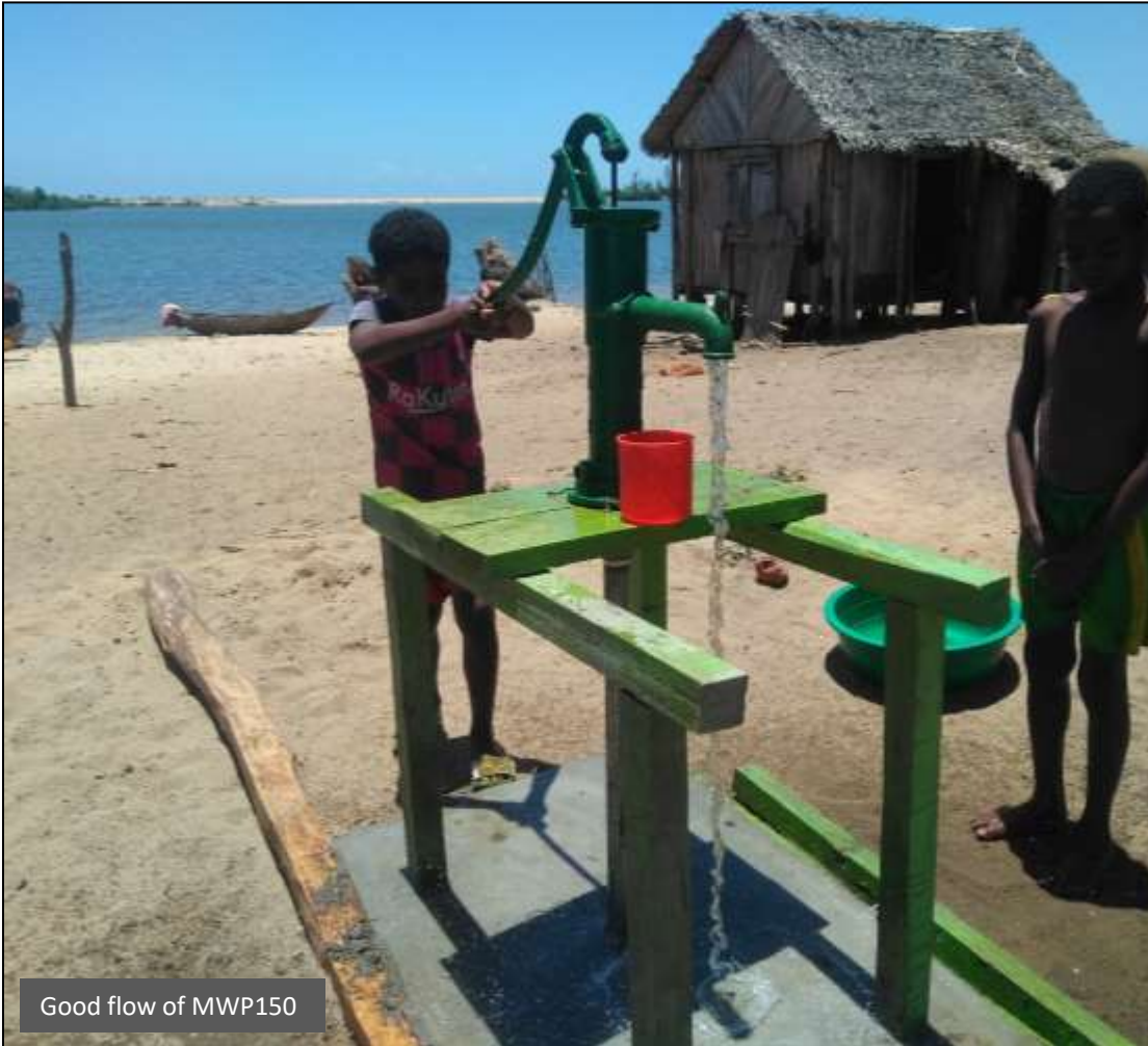
We did a coring, tried to put well point in a clear sand with a good reservoir
