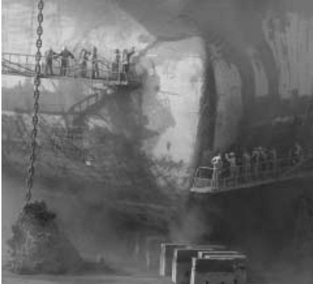
Fig. 1. Grit-blast crew at work.
