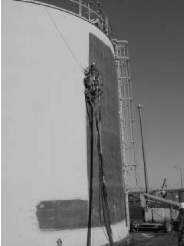
Fig. 6. M2000 stripping a storage tank.
