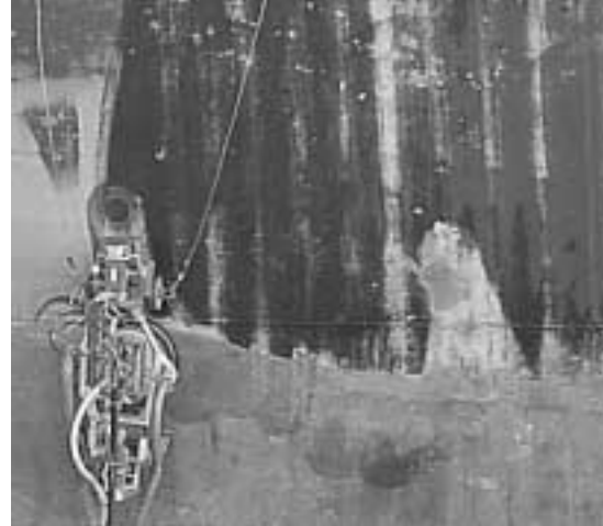
Fig. 8. Mottled surface after sweeping.
