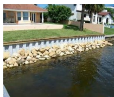
Vinyl Seawall with Rip Rap
