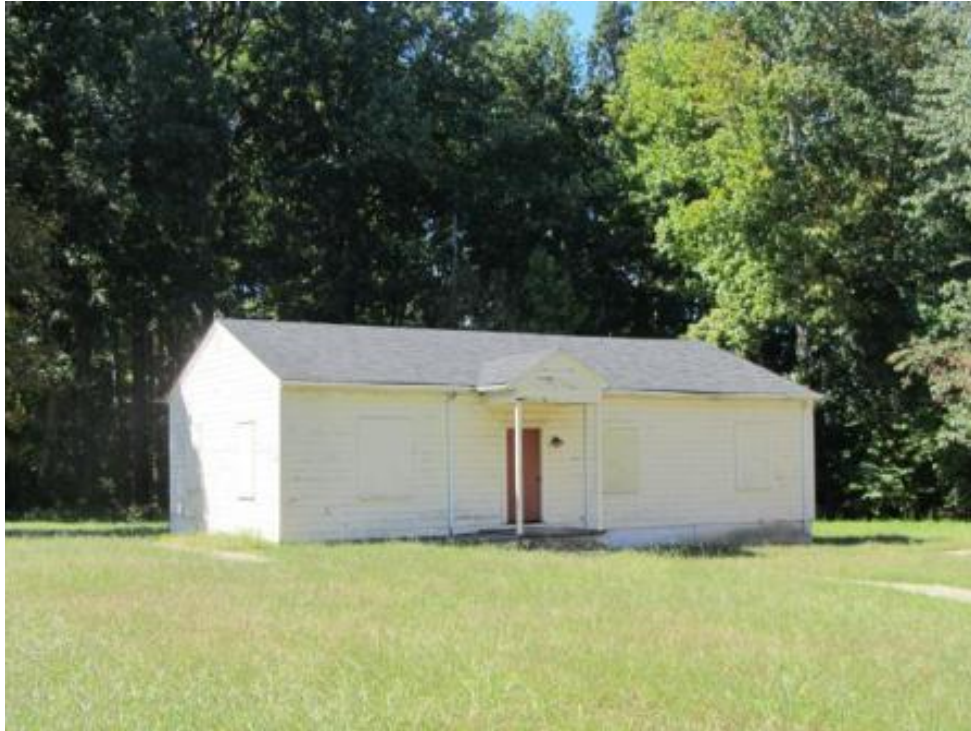
Figure 11. NCDOT Survey #41, Palmer Memorial Institute Historic District (GF-0180), Bryce-Maye Cottage, north elevation, looking south from in front of Reynolds Hall (Resource 1S on the site plan [see Figure 3]).
