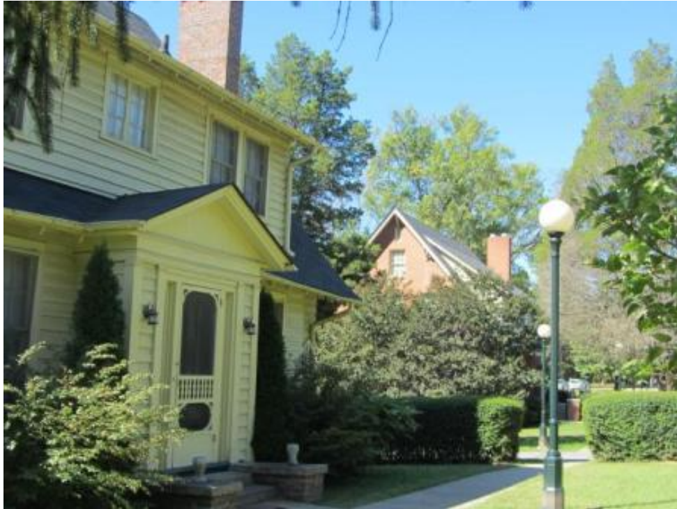
Figure 7. NCDOT Survey #41, Palmer Memorial Institute Historic District (GF-0180), view looking west from vicinity of Charlotte Hawkins Grave Site (south side of US 70) with Canary Cottage in foreground and Carrie Stone Cottage in background (Resources 1M and 1N respectively on the site plan [see Figure 3]).
