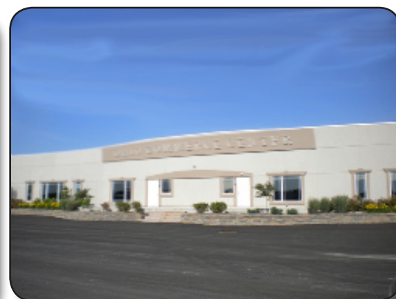
A partnership among the Chamber, Ohio Commerce Center and ms consultants, inc. was awarded a $2 million Job Ready Site Grant for rail, road and bridge work at the OCC industrial site in Lordstown.
